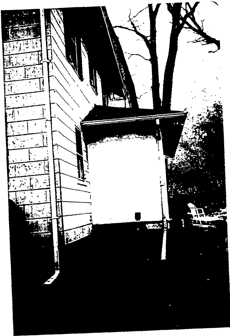
Rear of 10922 from North
