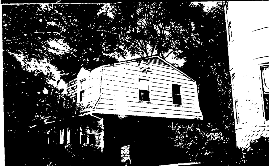
South side of our house.
