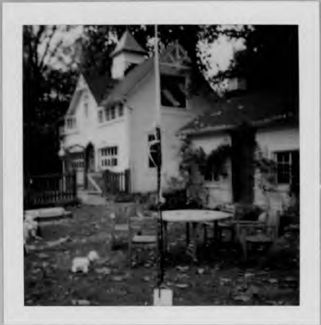
SHED & CARRIAGE HOUSE FROM EAST
