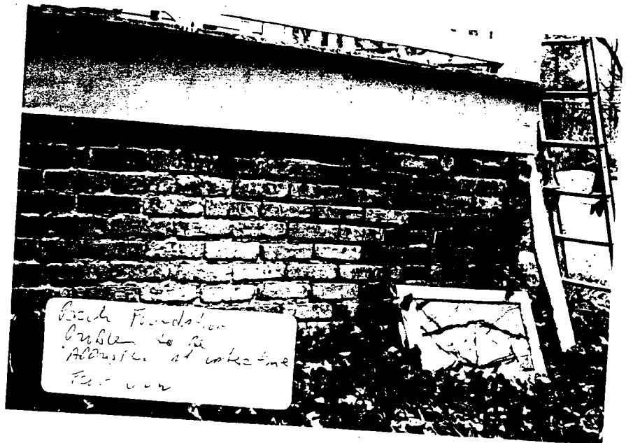
Side view Porch Foundation
