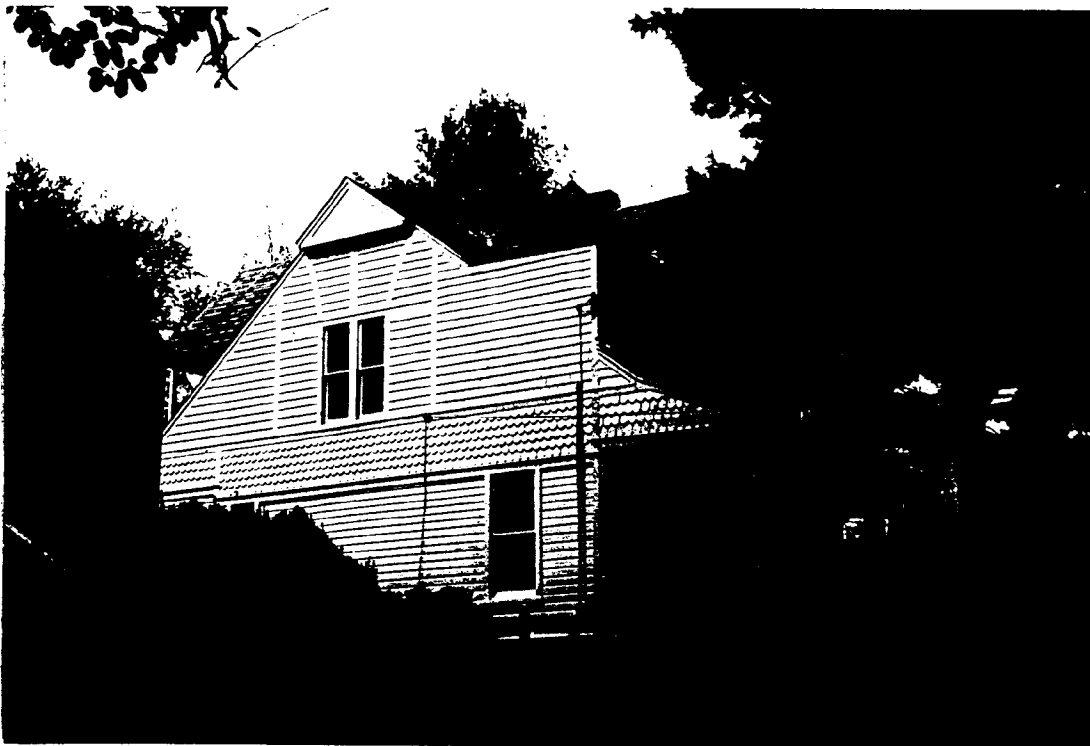
VIEW FROM KESWICK ST. SHOWING SOUTH ELEV. AND NEIGHBORING HOUSES
