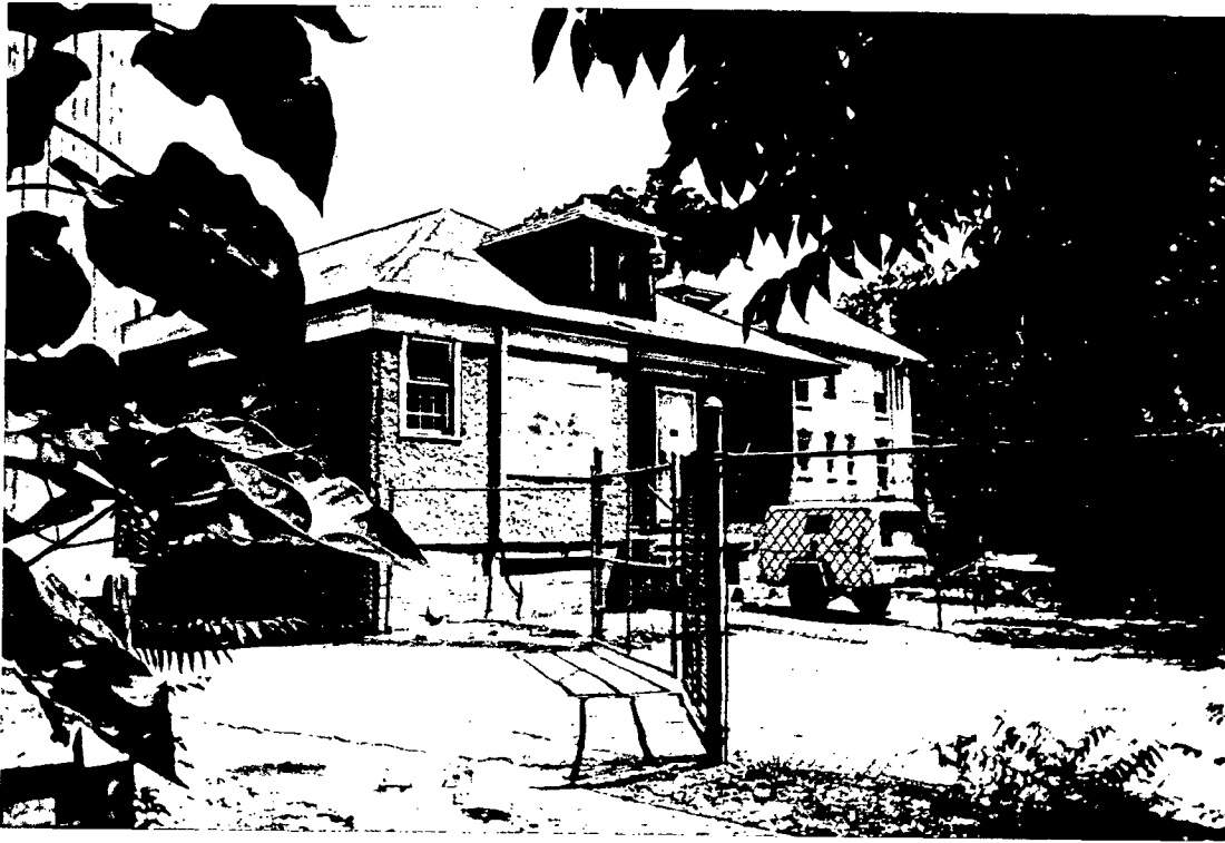
Rear of property. Chain link fencing shown to be removed. Fence will remain from face of garage to rear right corner of lot. Deck/platform shown at top of stairs will be replaced and extended to left edge of building (under window) to accommodate compressors.
