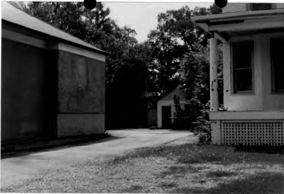
View of right side of building from front of 7063 Carroll Ave.
