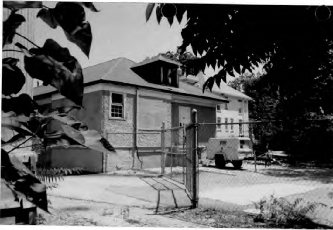
Rear of property. Chain link fencing shown to be removed. Fence will remain from face of garage to rear right corner of lot. Deck/platform shown at top of stairs will be replaced and extended to left edge of building (under window) to accommodate compressors.
