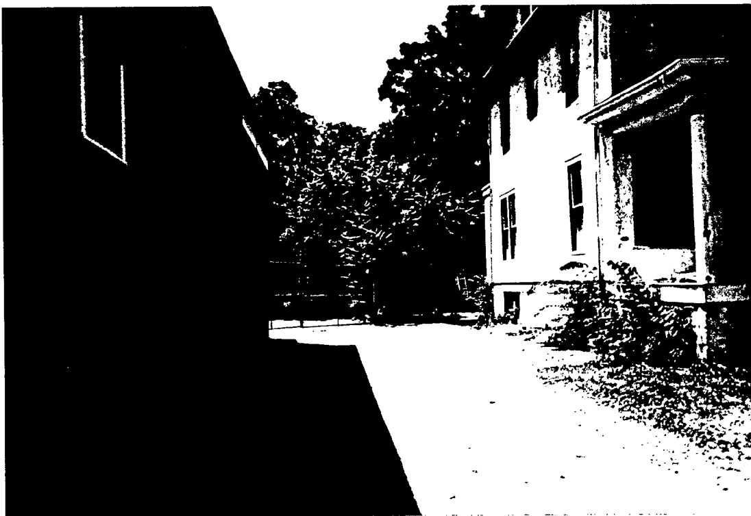
View of right side of building from front. One or two windows to be restored. Chain link gate to be removed.
