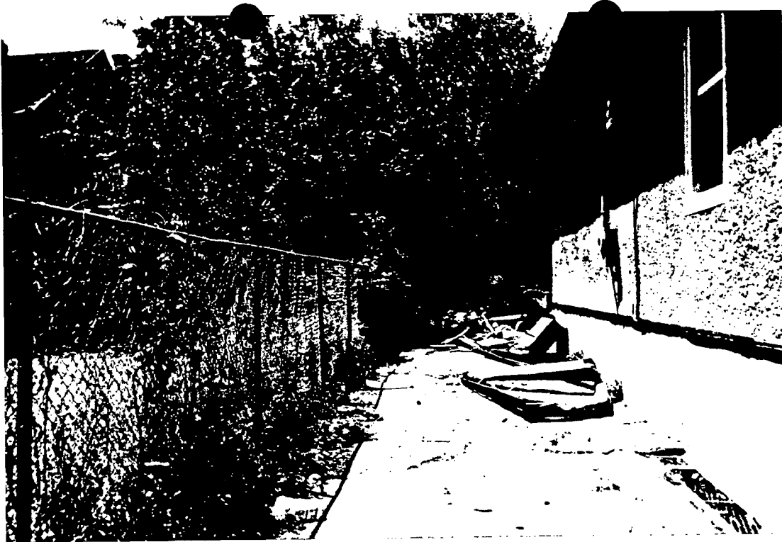
View of left side of building adjoining 1 Columbia Ave. Fence to be replaced by 6' wood. One or two windows to be restored.
