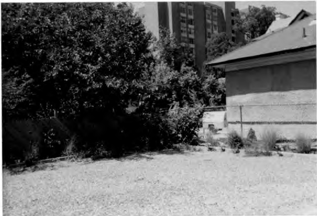
View of left side/rear from parking area of 1 Columbia Ave. Fence to be replaced by 6' wood.
