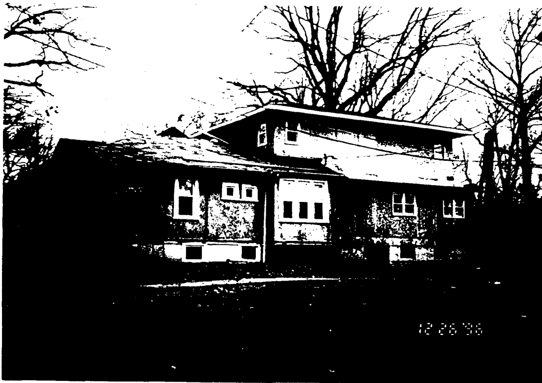
South Facade Facing Cleveland
