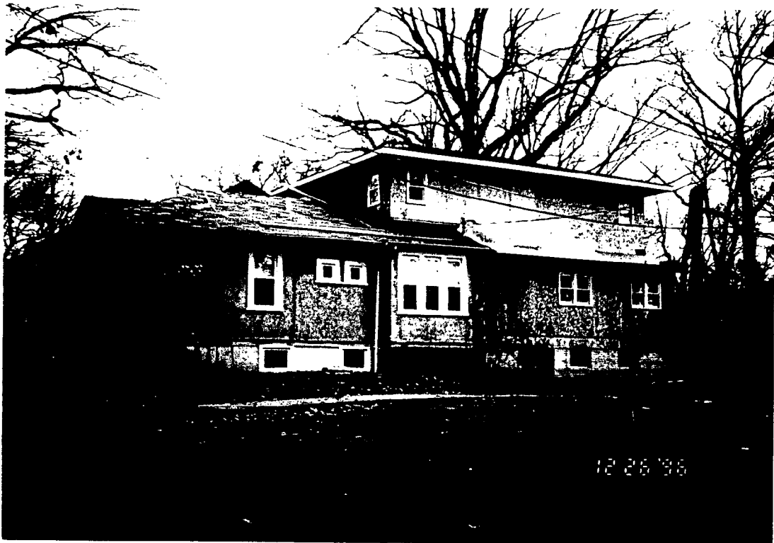
South Facade Facing Cleveland
