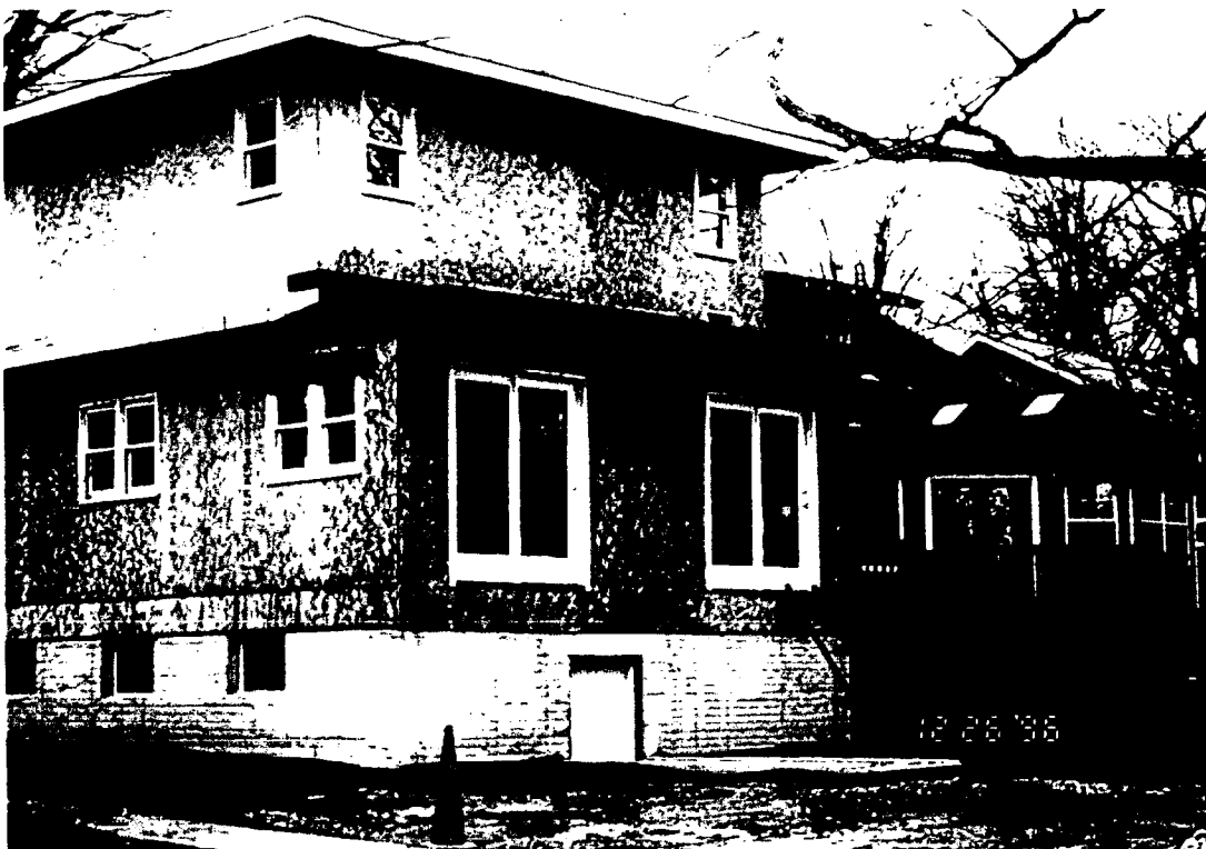
SE corner of New Addition (Rear)
