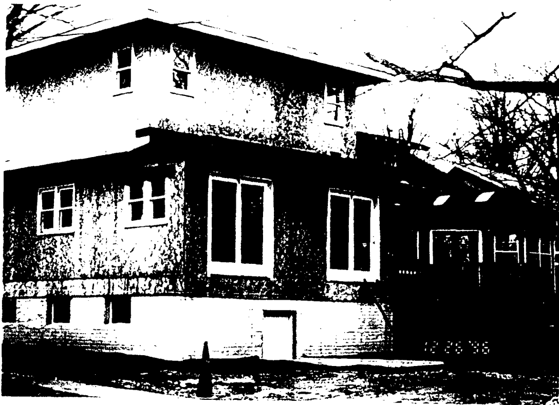
SE corner of New Addition (Rear)
