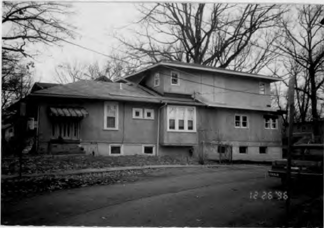
South Facade Facing Cleveland
