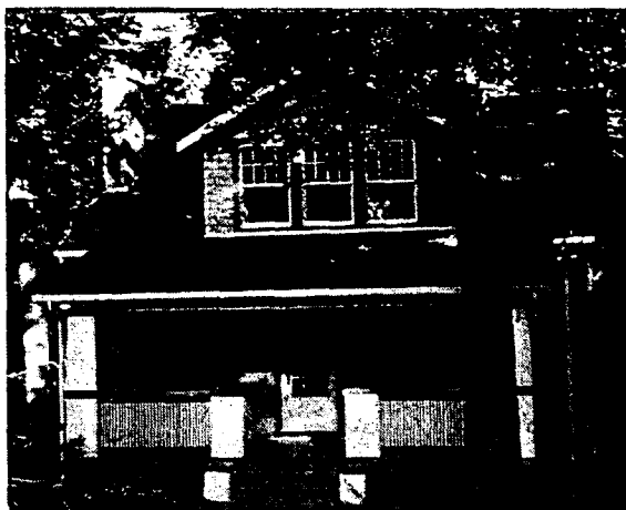
Example of a compatible alteration: An undersized non-historic dormer was replaced by the dormer shown which is more typical of Bungalows in Takoma Park.
