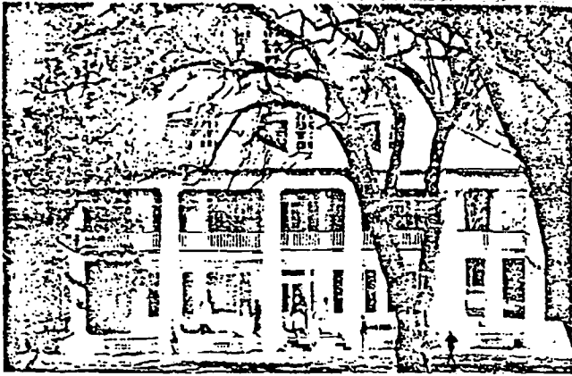
Figure 3. Southern mansions typify climate conscious design. The wide roof overhangs, exterior porches, shade trees, heavy masonry walls (painted white), and living quarters on the second floor (to catch evening breezes and escape the radiant heat from the earth's surface) all are energy saving characteristics which provide reasonably comfortable living spaces without mechanical air conditioning. (Photo: Marcia Axtmann Smith)
