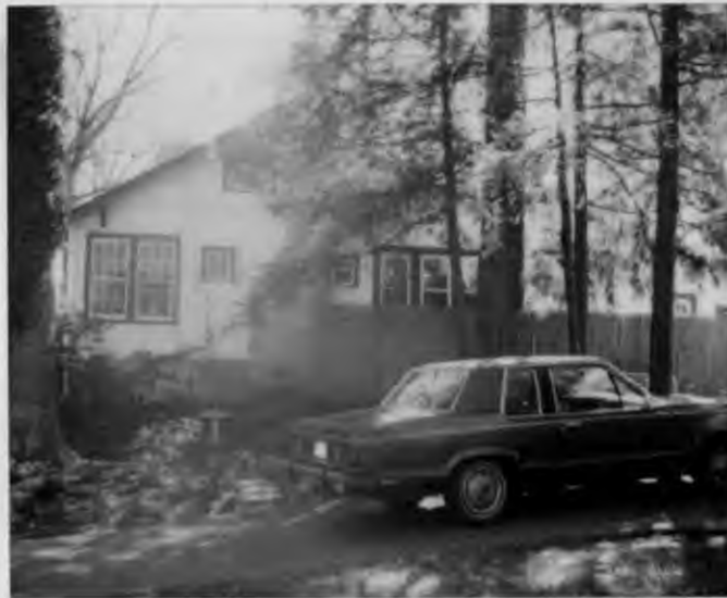
Silver Renovation 7324 Baltimore Ave., Takoma Park ② Window to be removed 3-17-88
