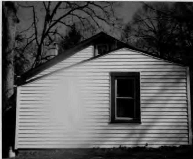
Silver Renovation 7324 Baltimore Ave., Takoma Park ③ New door & window to be added 3-17-88
