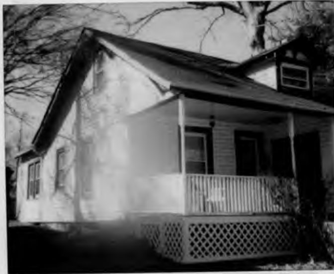
Silver Renovation 7324 Baltimore Ave., Takoma Park ④ New dormer to be added at rear 3-17-88
