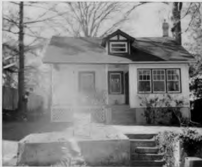
Silver Renovation 7324 Baltimore Ave., Takoma Park ① New brick pier and wood posts 3-17-88
