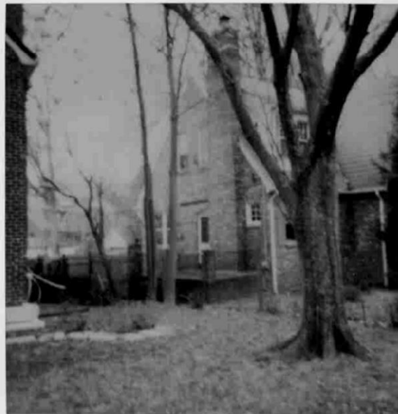
7441 Baltimore Ave Left Oblique ③
