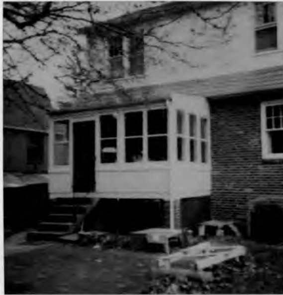
7441 Baltimore Ave Existing Rear Porch (6)
