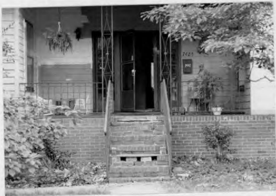
7425 Buffalo Ave Existing Steps
