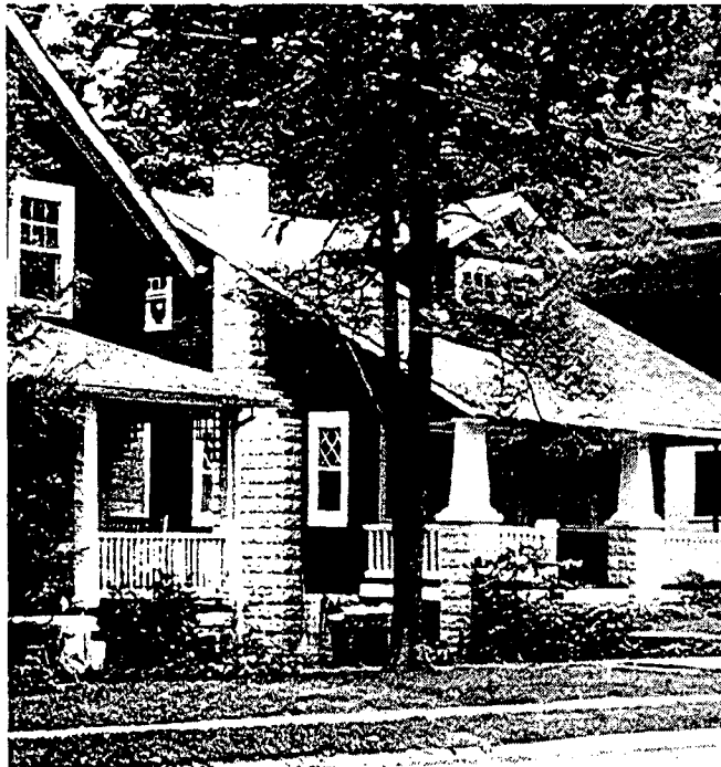
☒ Contributing resources on Hickory Avenue
