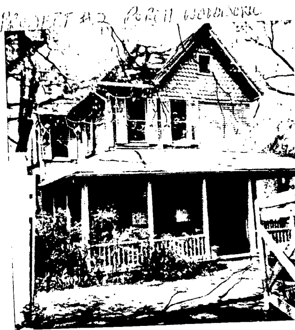
Milmoe 7212 Cedar Ave, Tk, Pk, Md view from Cedar Ave.
