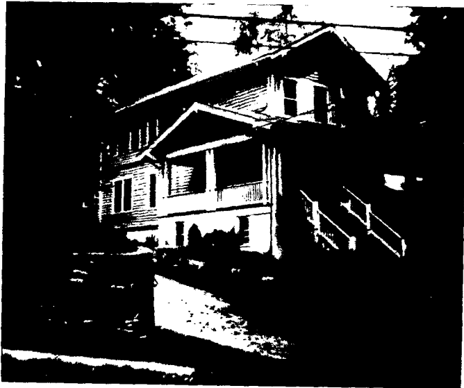
VIEW OF SOUTHWEST AND SOUTHEAST (FRONT) SIDES OF HOUSE
