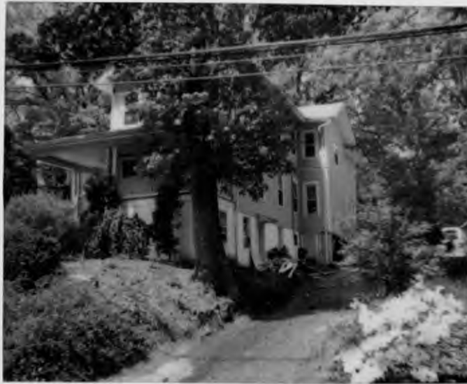
VIEW OF NORTHEAST SIDE OF HOUSE
