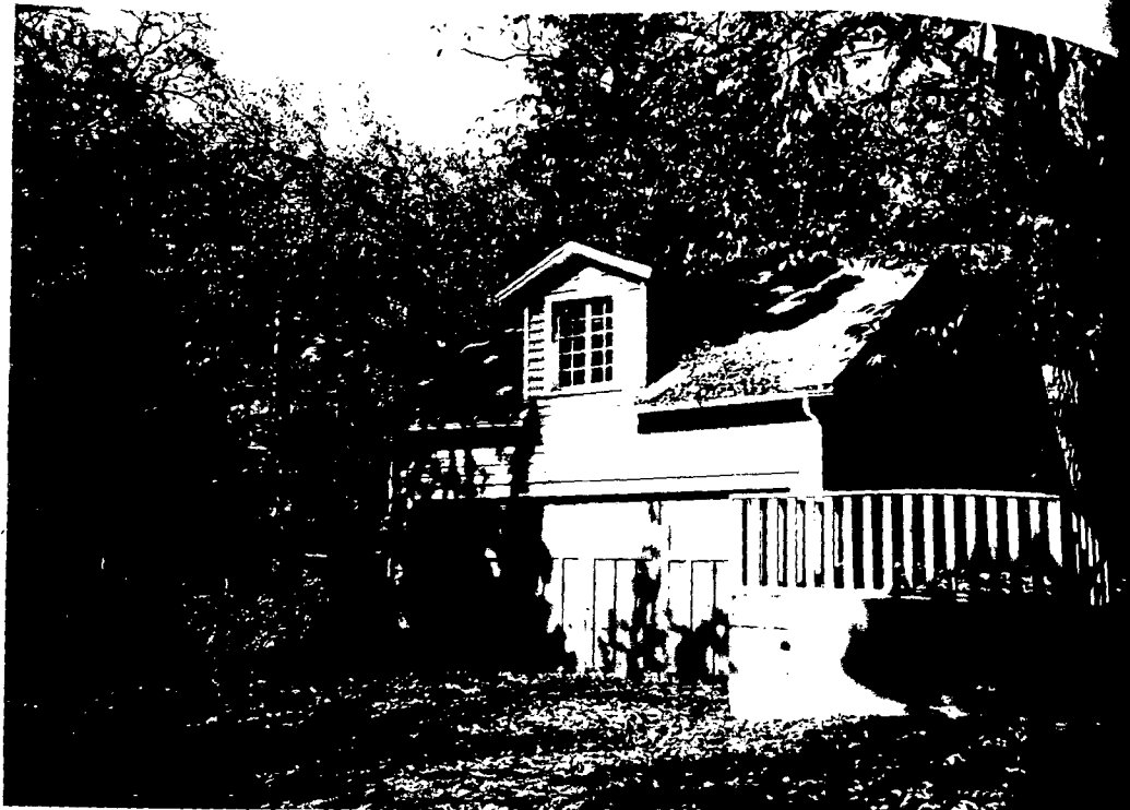
GARAGE - FRONT / RIGHT SIDE (SOUTH EAST CORNER)
