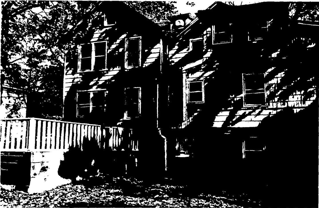
MAIN BUILDING - REAR VIEW (WEST)
