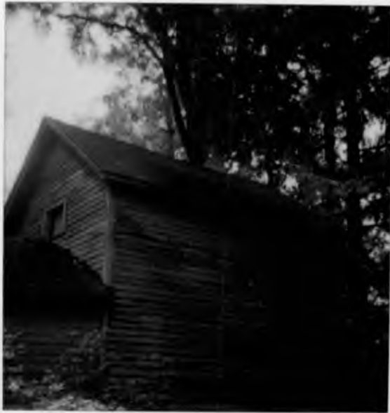
Carriage House Existing Condition
