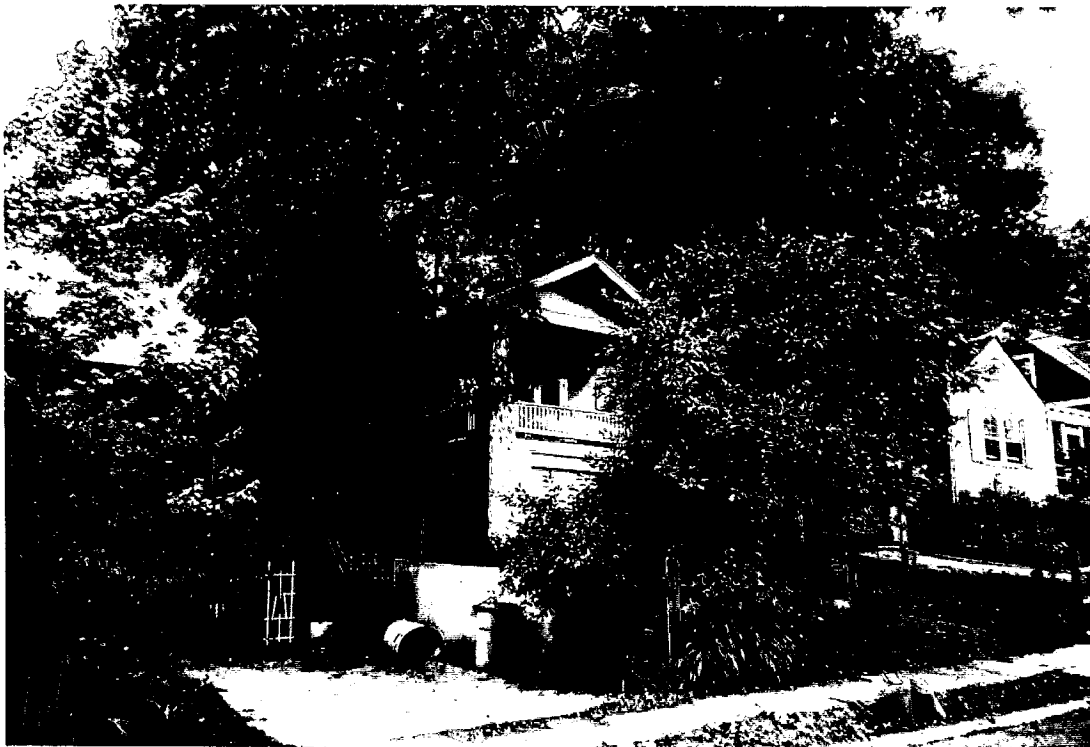
PHOTO A-4: Exterior West Elevation
