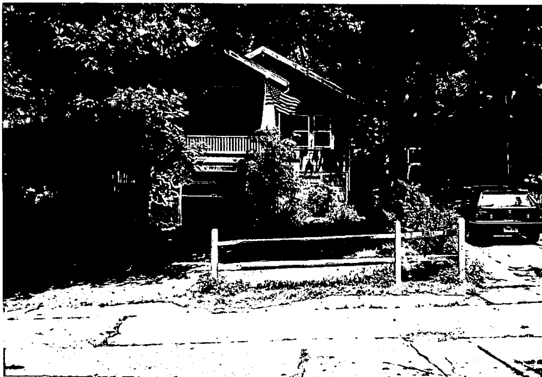
PHOTO A-1: Exterior South Elevation
