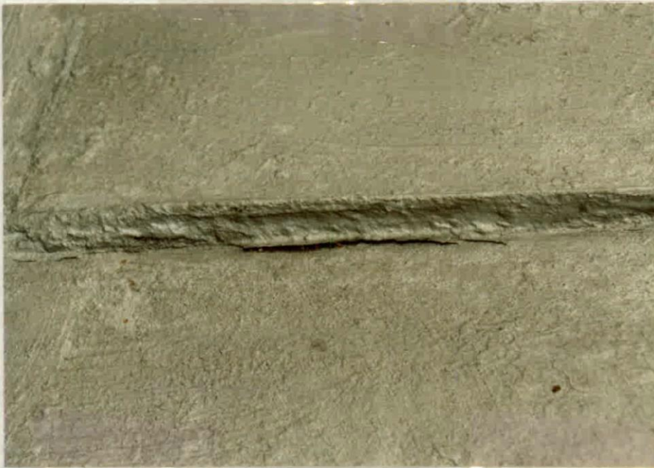
F. CLOSE UP OF STANDING SEAM
