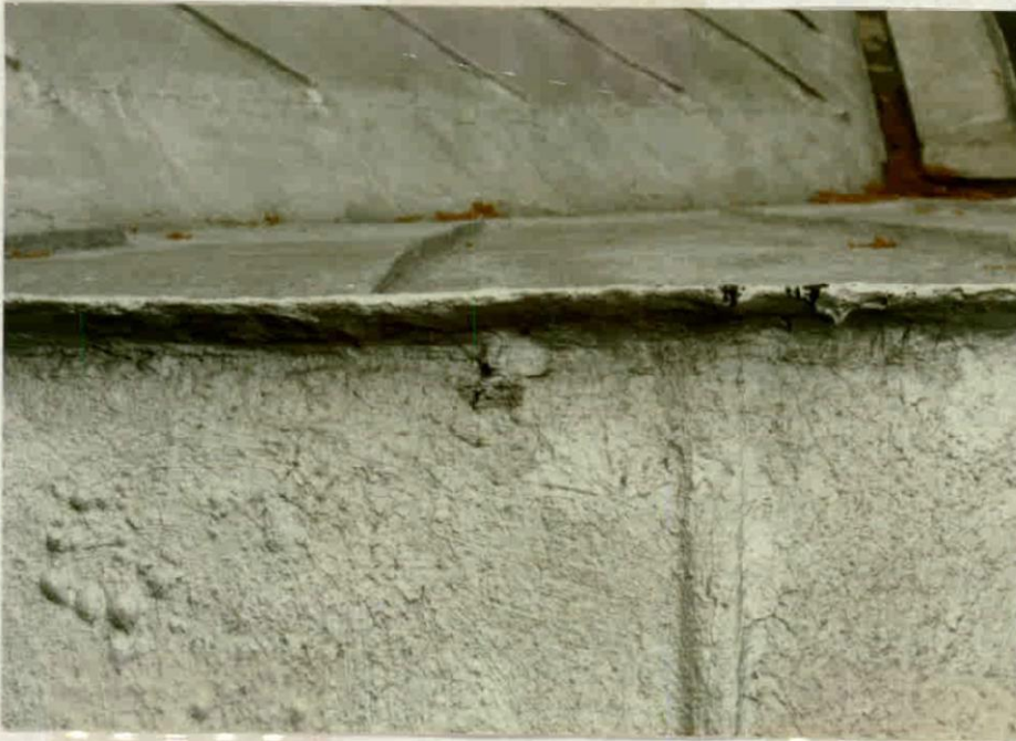
E. CLOSE UP OF STANDING SEAM
