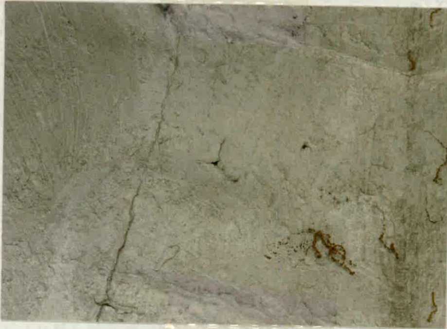
G. CLOSE UP OF TIN ROOF SURFACE
