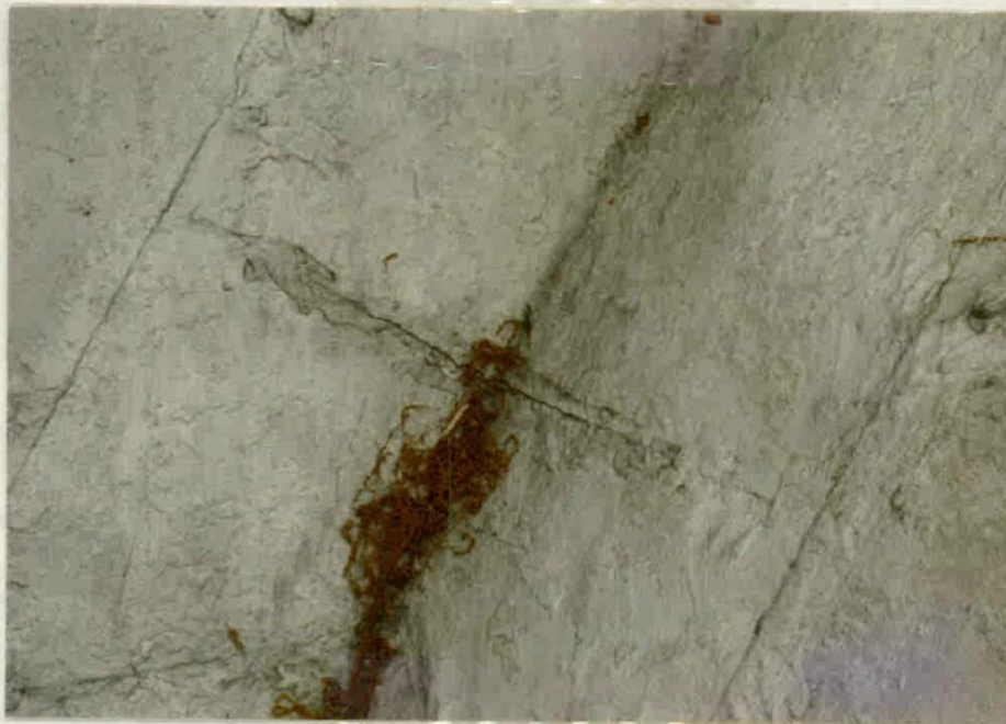
H. CLOSE UP OF TIN ROOF SURFACE
