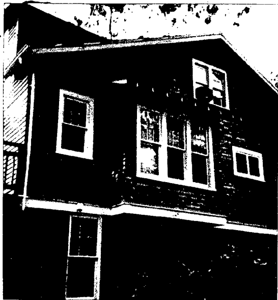
SIDE VIEW WHERE WORK WILL TAKE PLACE
