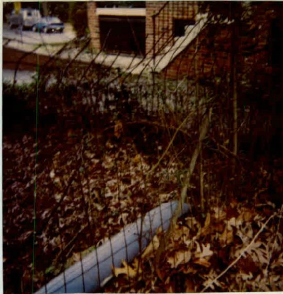
DETAIL OF WIRE MESH ON LEFT SIDE OF HOUSE BEING replaced
