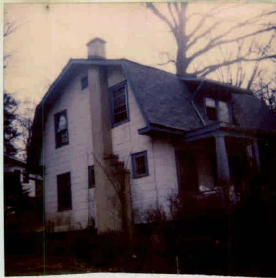
LEFT SIDE Replacing wire mesh where old is.
