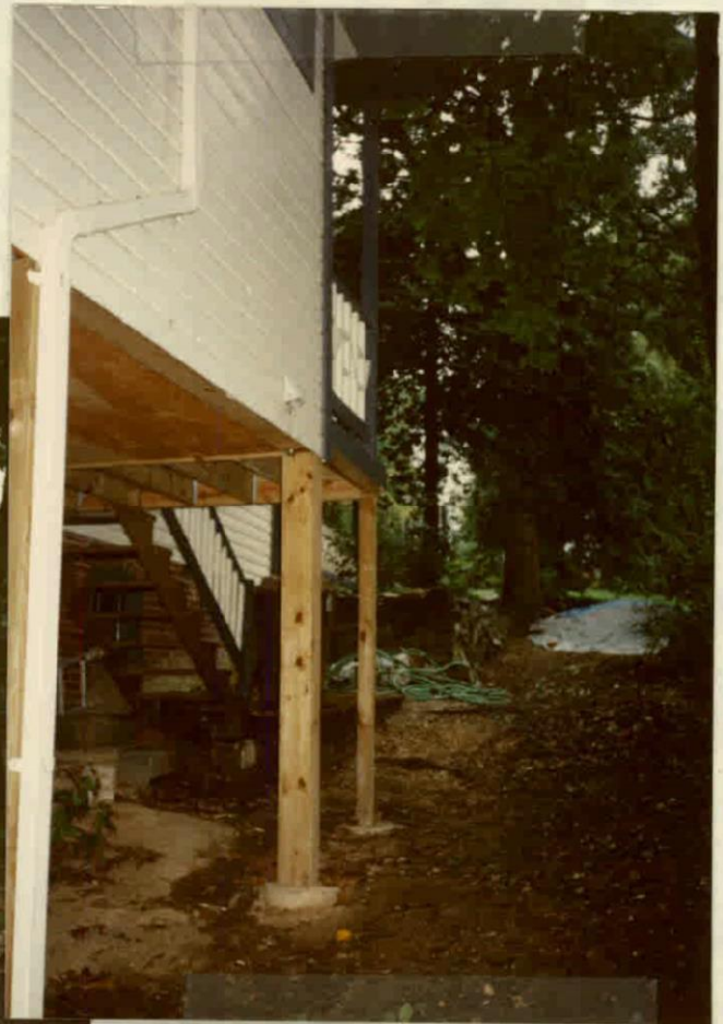
DRIVEWAY FACING STREET
