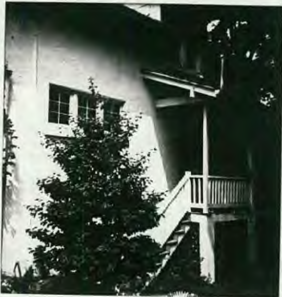
Right side - southeast showing existing side porch
