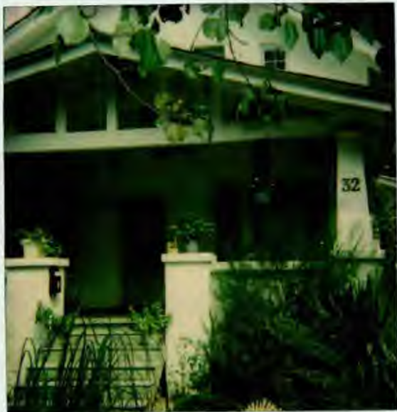
Front At Sidewalk 32 Philadelphia Ave
