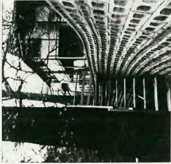
Back of main building
