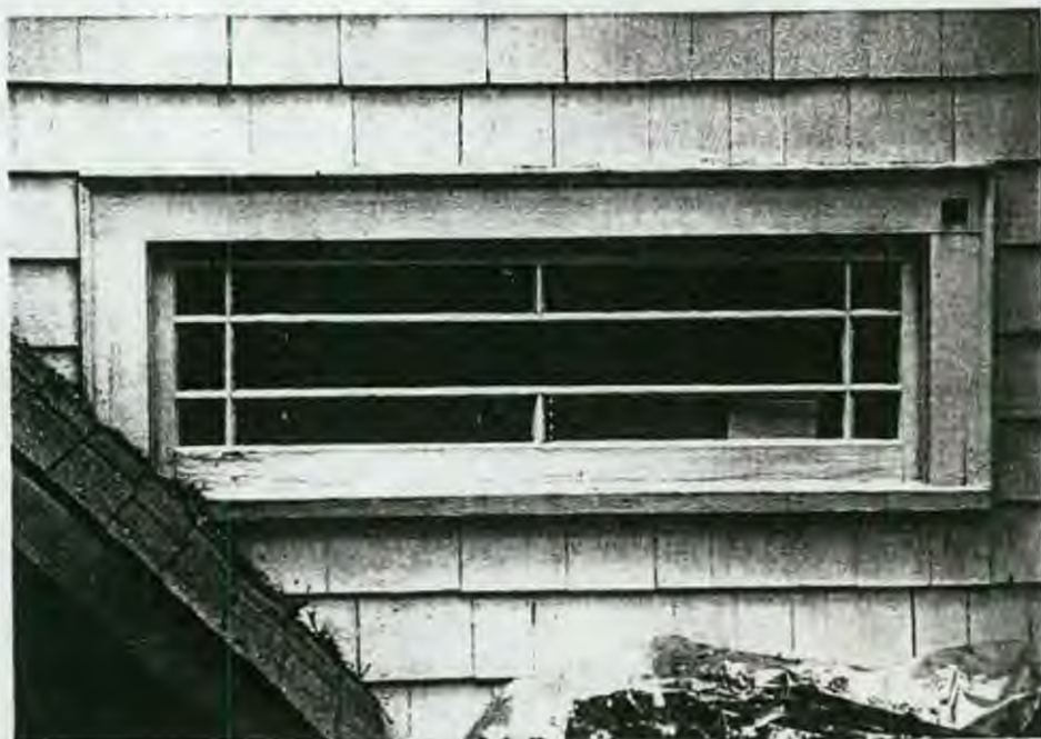
DETAIL OF DINING ROOM WINDOW
