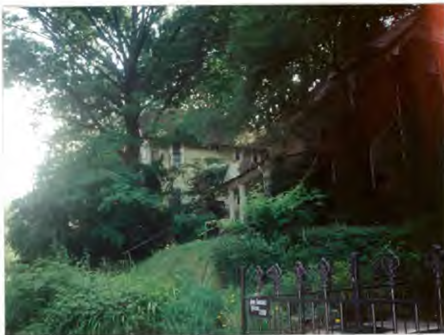
NORTHEAST SIDE OF 7410 PINEY BRANCH ROAD. PHOTO TAKEN FROM PINEY BRANCH ROAD.
