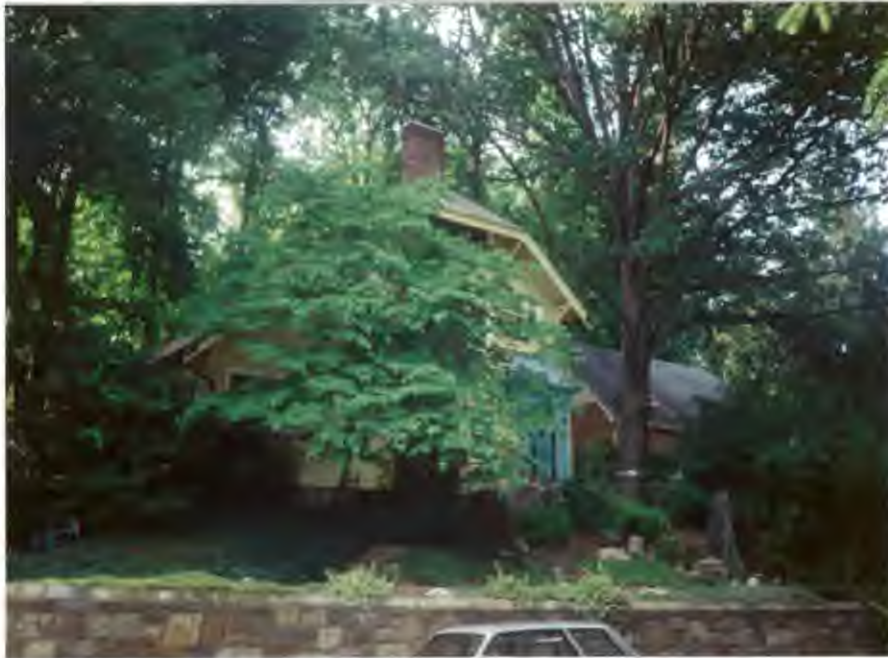
FRONT SOUTHEAST ELEVATION OF 7410 PINEY BRANCH ROAD. PHOTO TAKEN FROM SOUTHEAST SIDE OF PINEY BRANCH ROAD.
