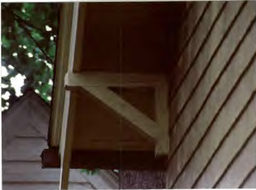
ROOF BRACKETS DETAIL
