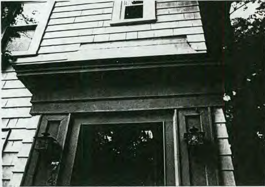
ENTRY CORNICE W/COPPER ROOF
