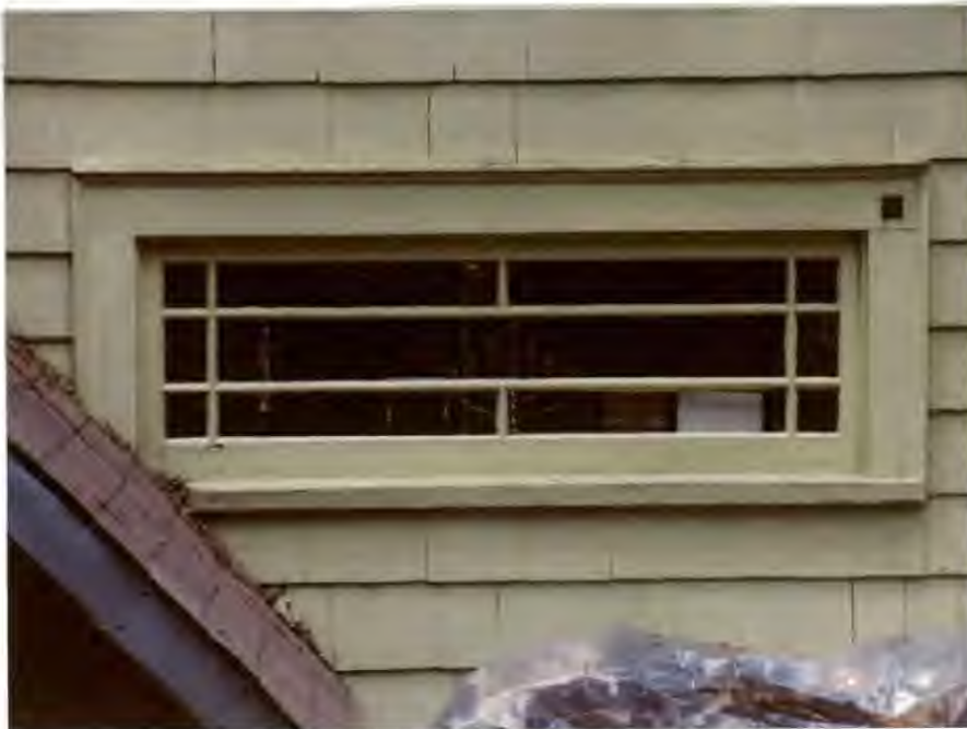
DETAIL OF DINING ROOM WINDOW
