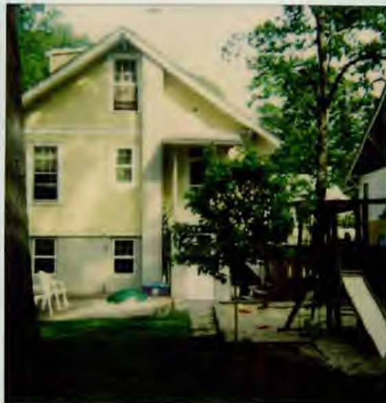
View of back of house Porch to be built off of 1st Floor (not basement) door.
