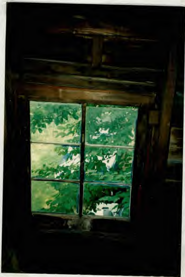
(40) View out of west window on second floor.
