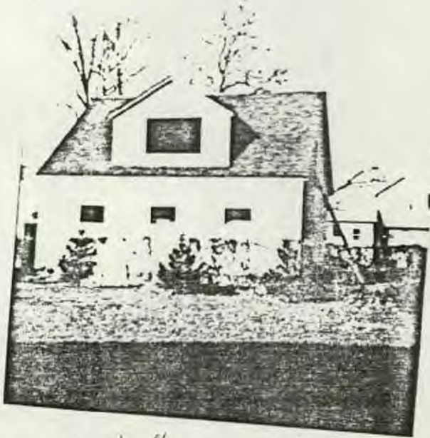
partially completed garage
