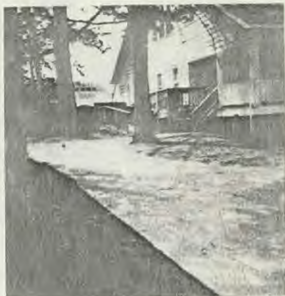
View of ramp from sidewalk
