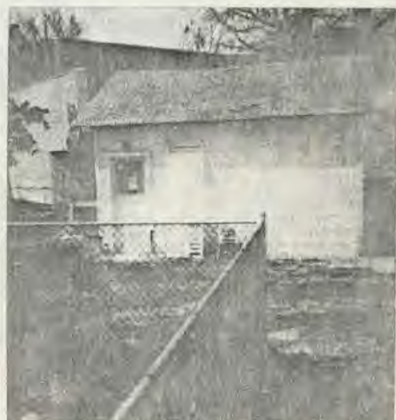
View of left side of garage
