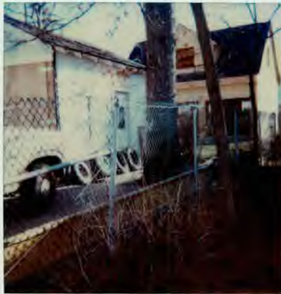
View of left side from old garage
