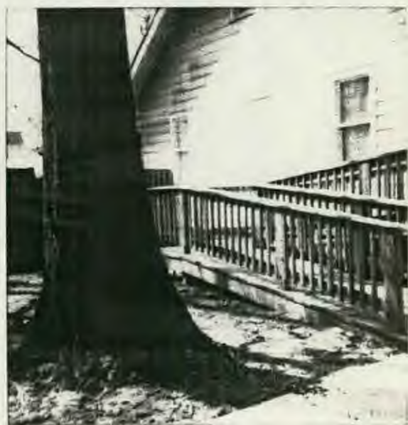
Close up of ramp and window
