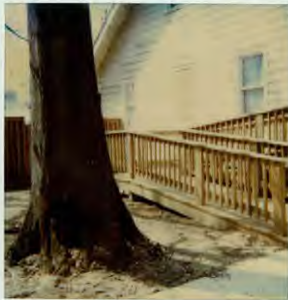
Close up of ramp and window
