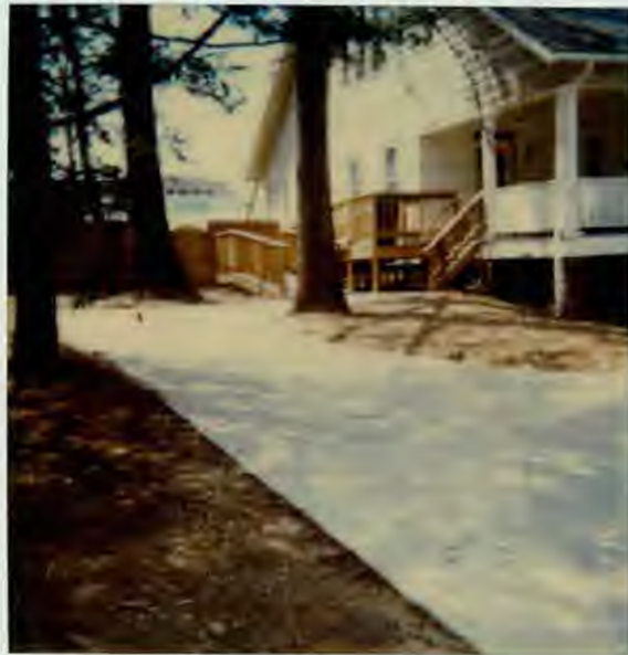
View of ramp from sidewalk
