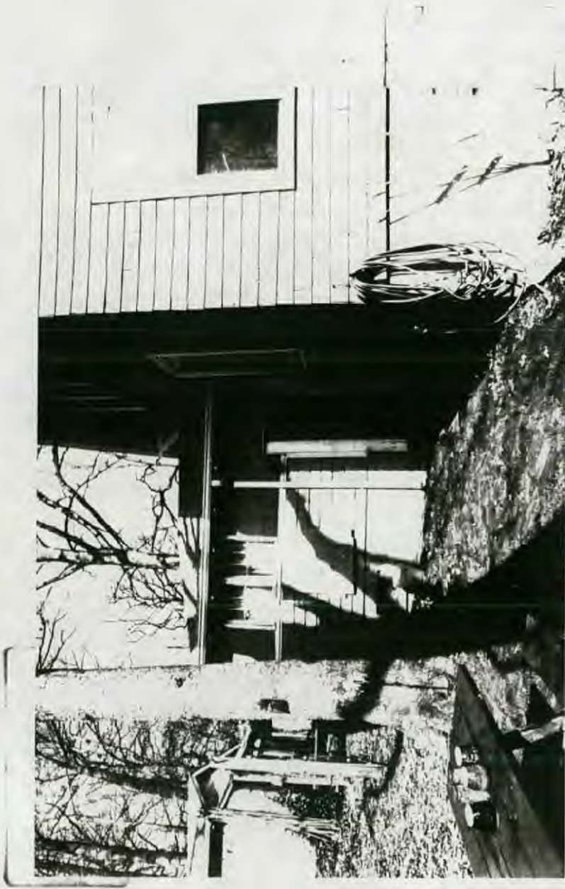
View from S.E. showing current 1-story addition & proximity of Oak tree.
