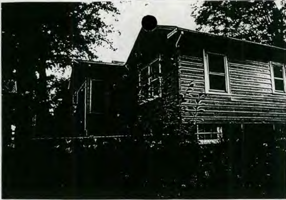
VIEW OF PROPOSED ADDITION AREA FROM BACK YARD OF 7213 WILLOW
