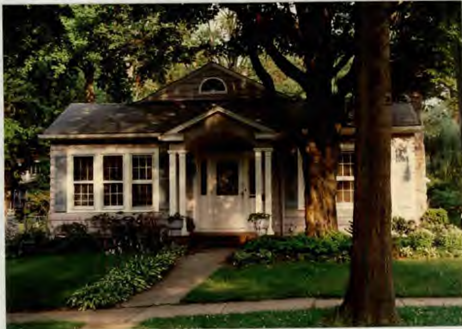
FRONT VIEW OF EXISTING RESOURCE
