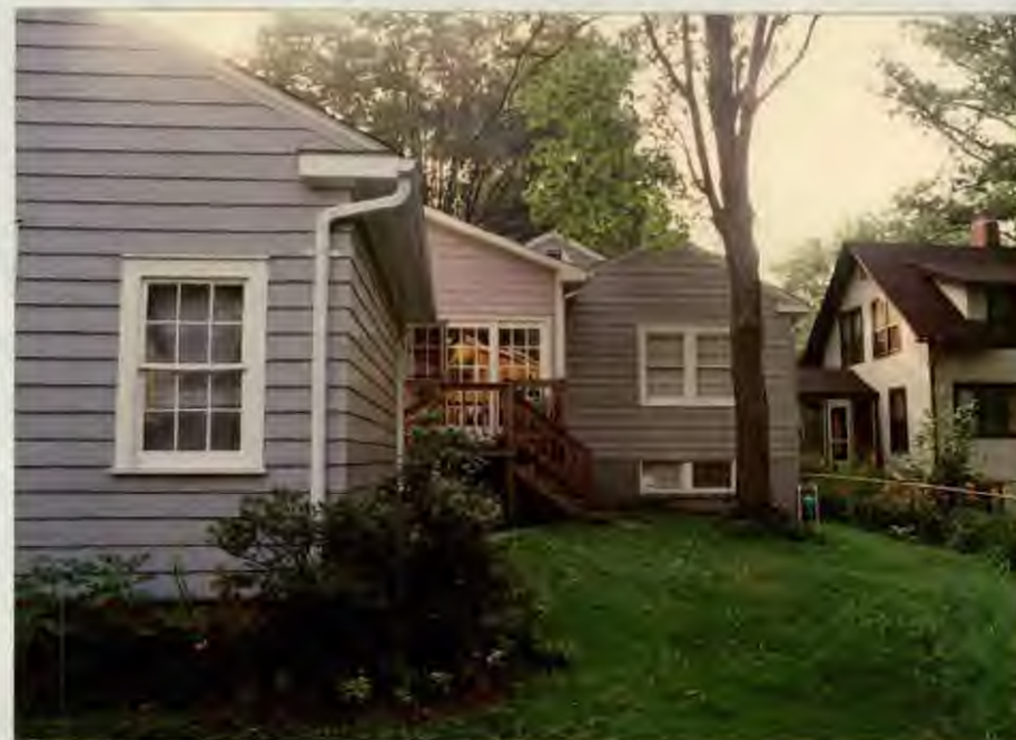
VIEW OF PROPOSED ADDITION AREA. DISEASED TREE WILL EITHER HAVE DECK BUILT AROUND OR WILL BE REMOVED - BASED ON CITY ARBORIST'S RECOMMENDATION.
