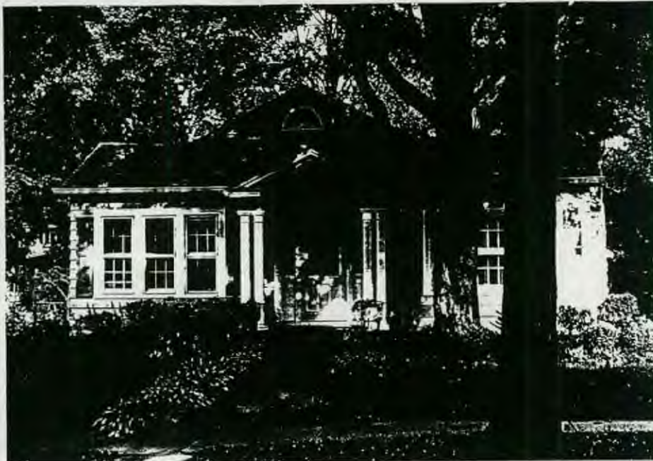
FRONT VIEW OF EXISTING RESOURCE
