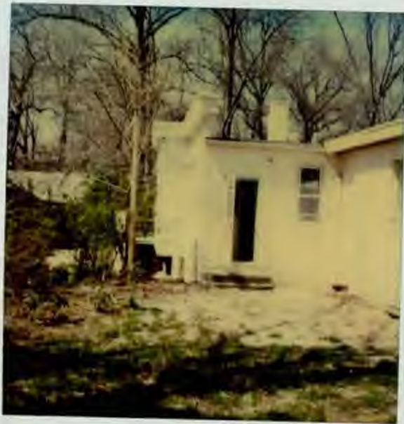
Rear view of 7315 Willow standing 214 shows the point where the deck will end. Deck height 6 inches below 2001 sill
