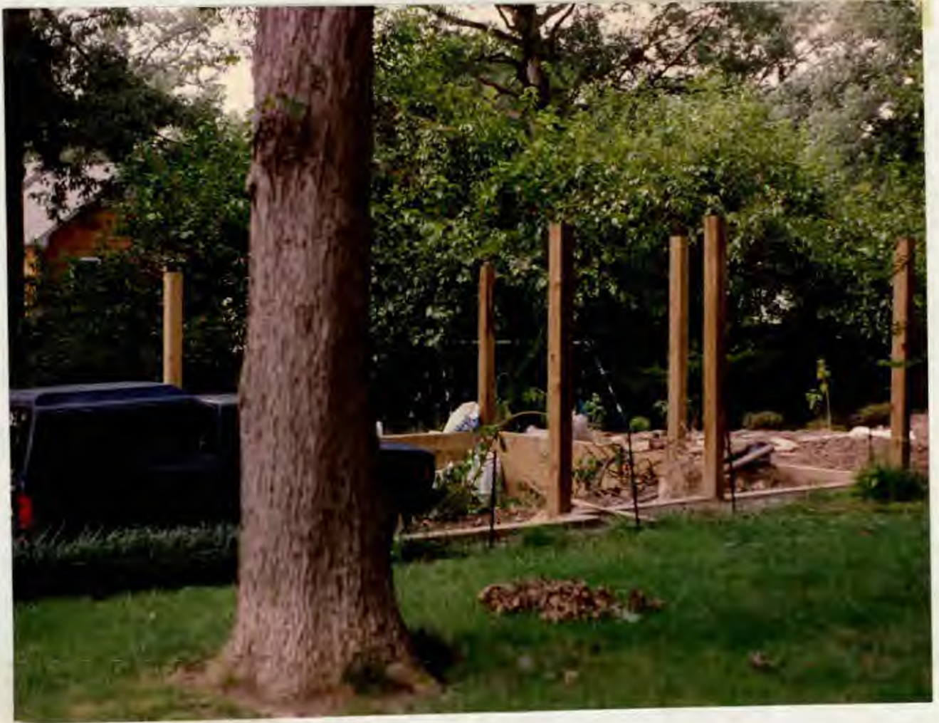
Photo of carport taken from the middle of my yard
