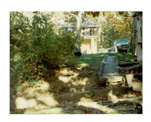
1. Area where brick retaining wall is proposed to be constructed to prevent soil exosion (visible) wall will replace existing coment wall (in picture) which is too low. Wall will run in approx. North-South direction (parallel to Sycamore Ave.) Wall is to run from steps to approx. Z'z At. short of Columbia Ave.
