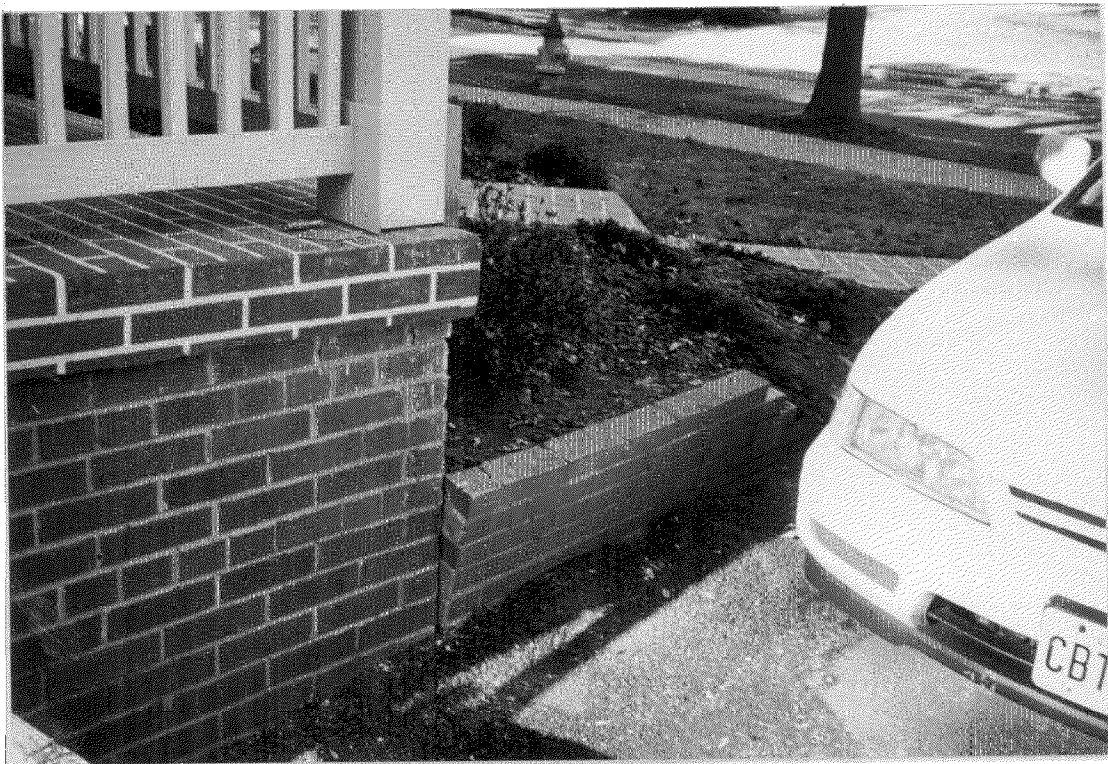
retaining wall - side view (BEFORE)
