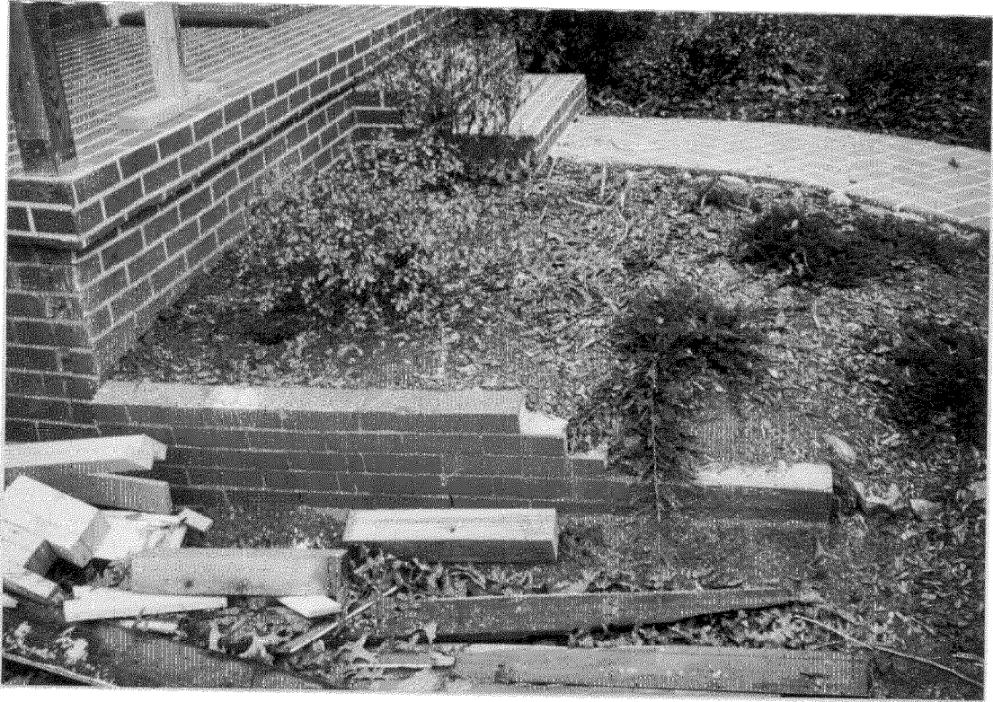
Existing retaining wall - Front side porch (Before)
