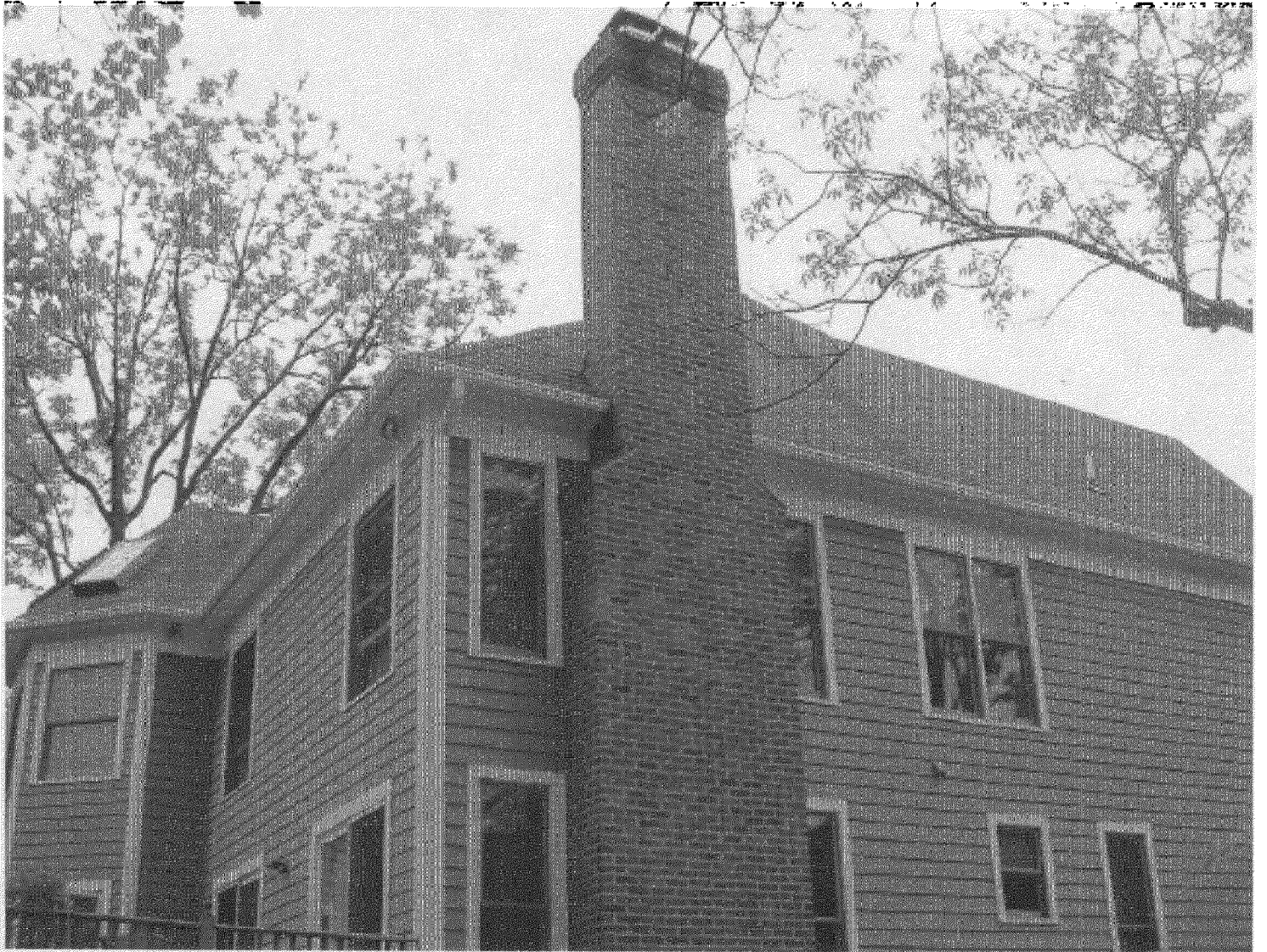
View of 10309 Freeman Pl. showing asphalt shingles similar to ones that will be used on 3824 Warner St.
