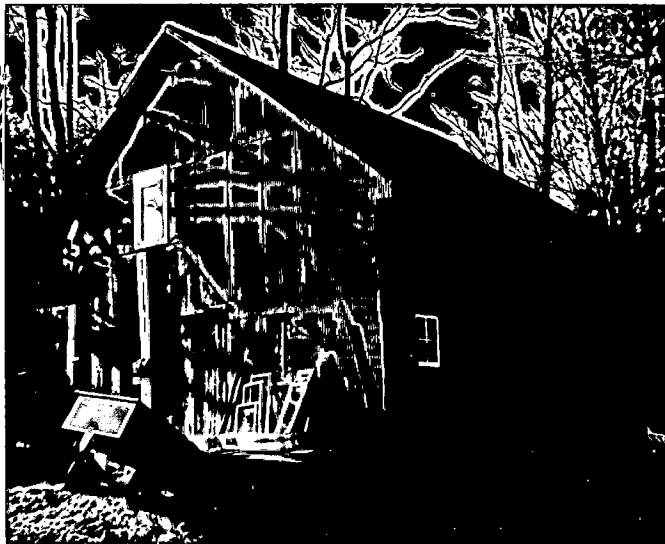
OUT BUILDING 25914 FREDERICK RD
