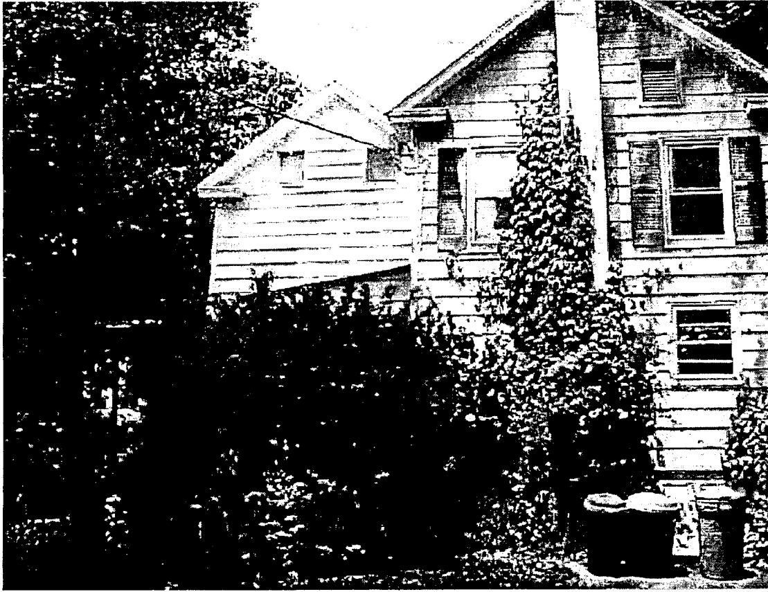
Side view of house Bushes will be removed.
