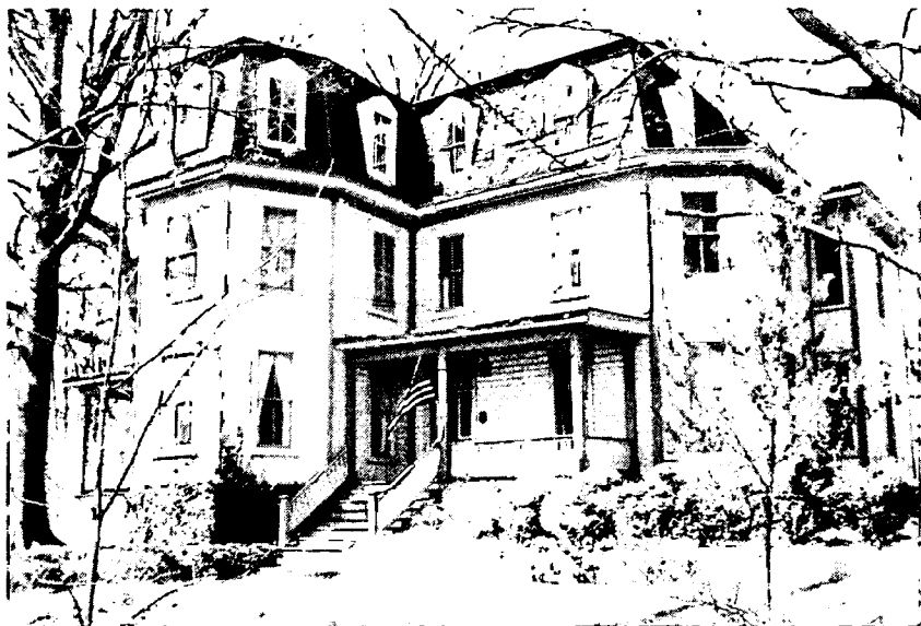
Historic High View contains 22 rooms set on nearly 5 acres.
