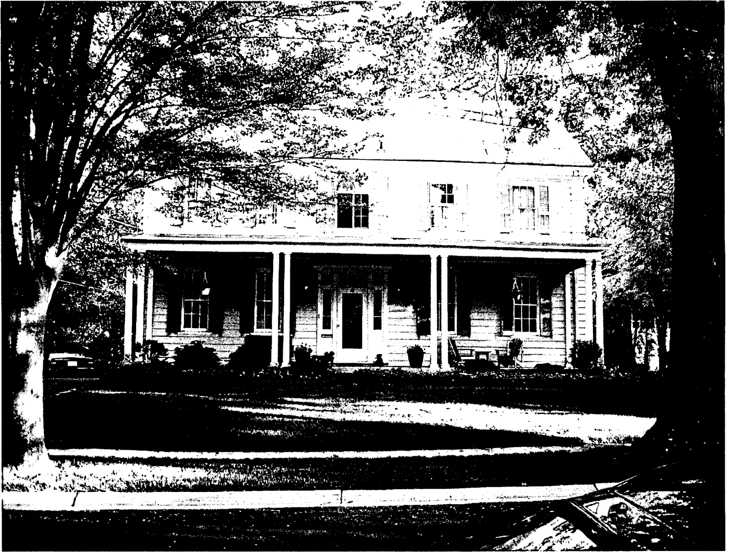
36 Quincy - existing conditions
