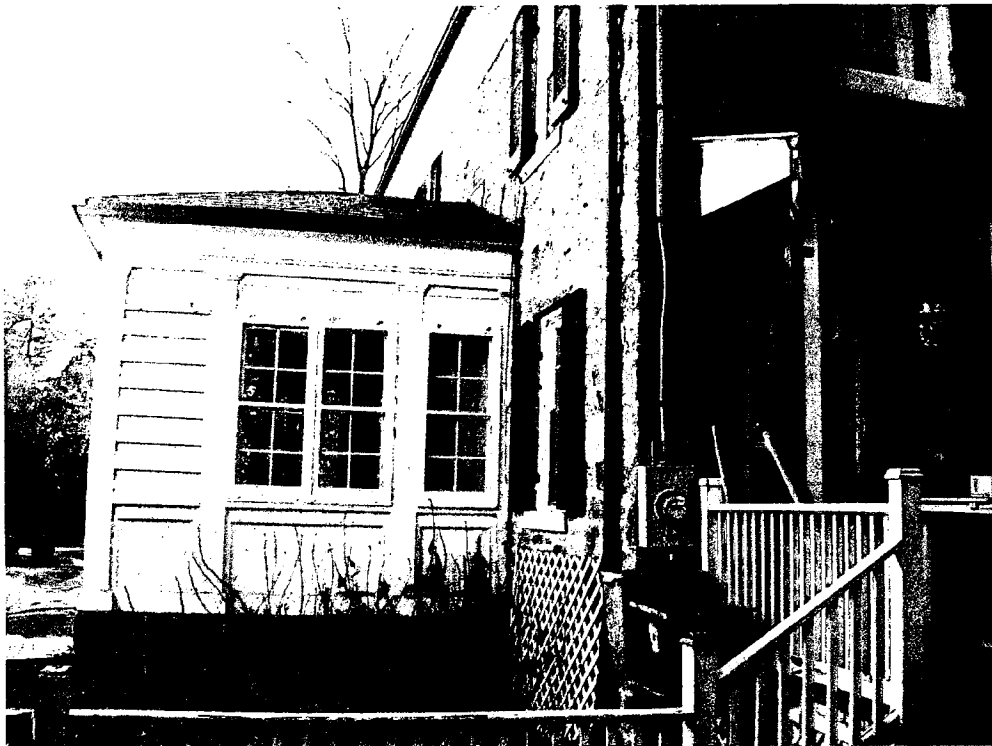
7 Primrose Street ---- Rear View of east side of house
