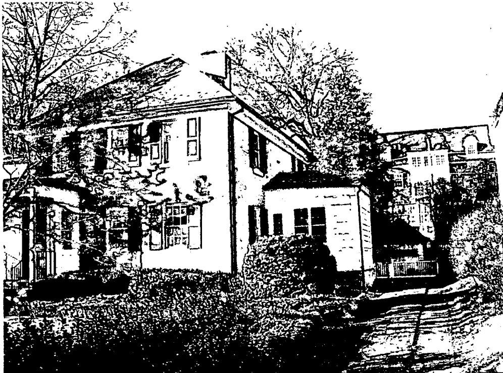
7 Primrose Street ---- Front View from SE corner
