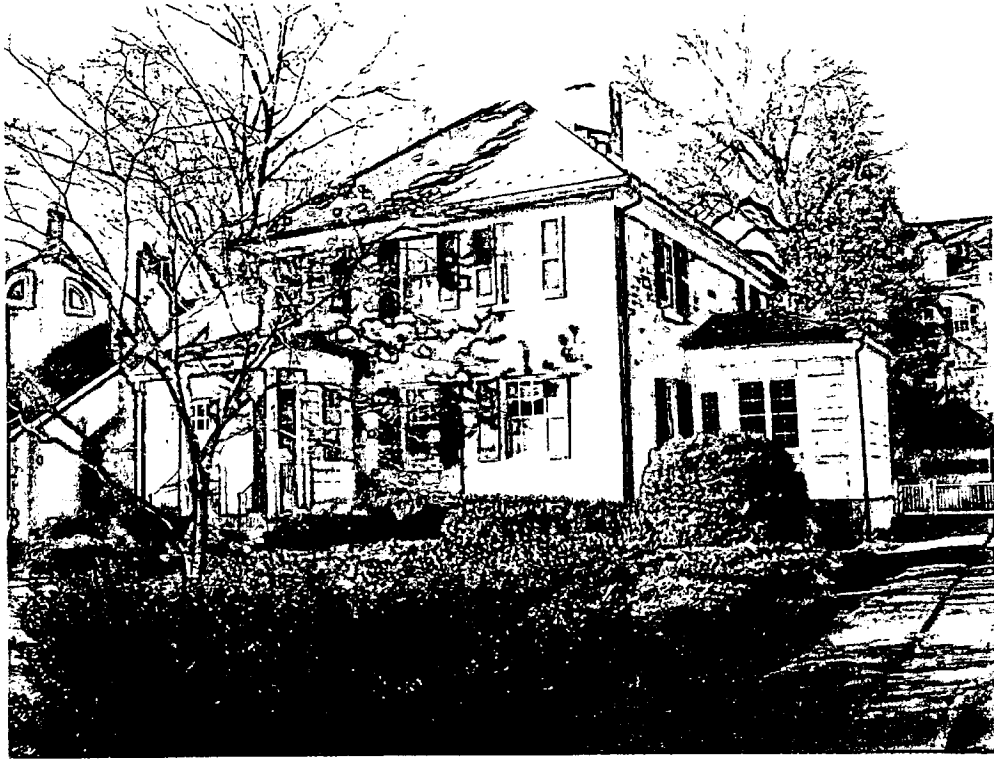
7 Primrose Street ---- Front View from SE corner
