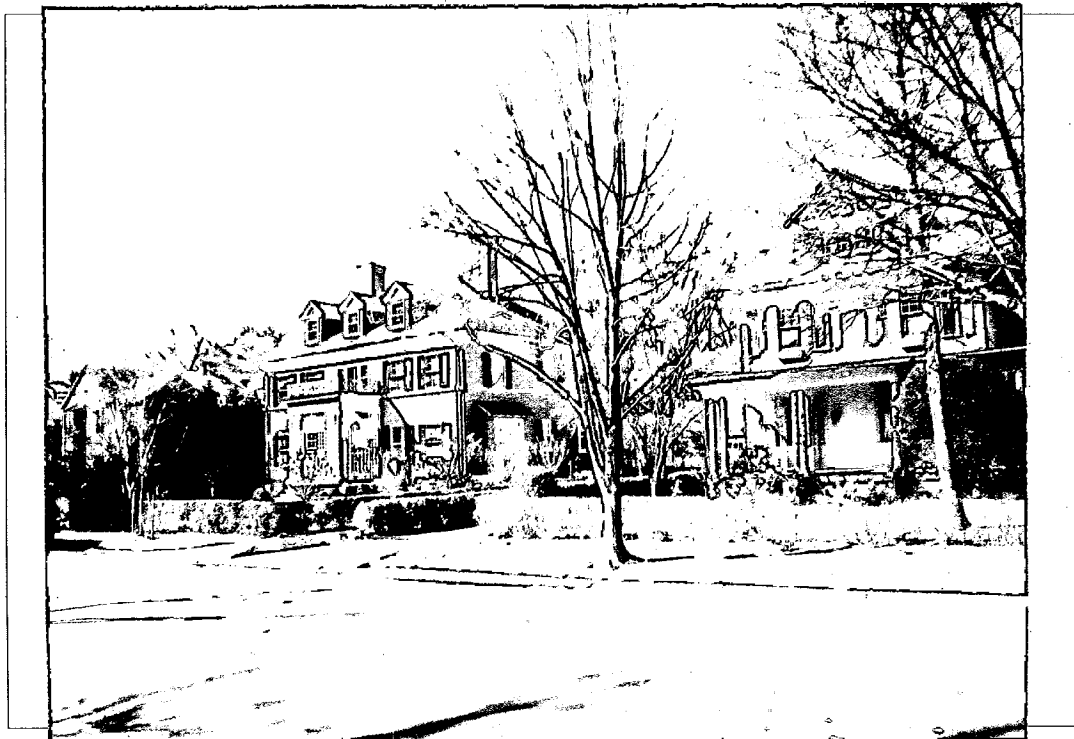
Detail: Primrose Street from #22 looking North West
