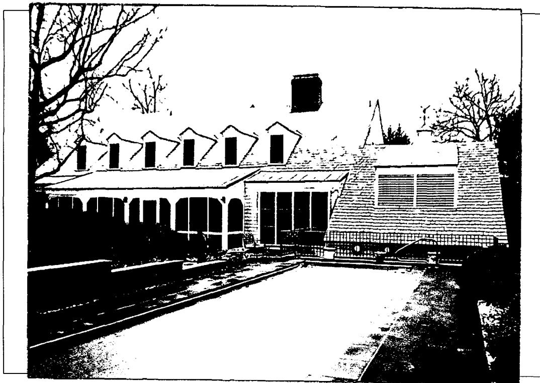
Detail: 22 Primrose St. (Rear) from South East
