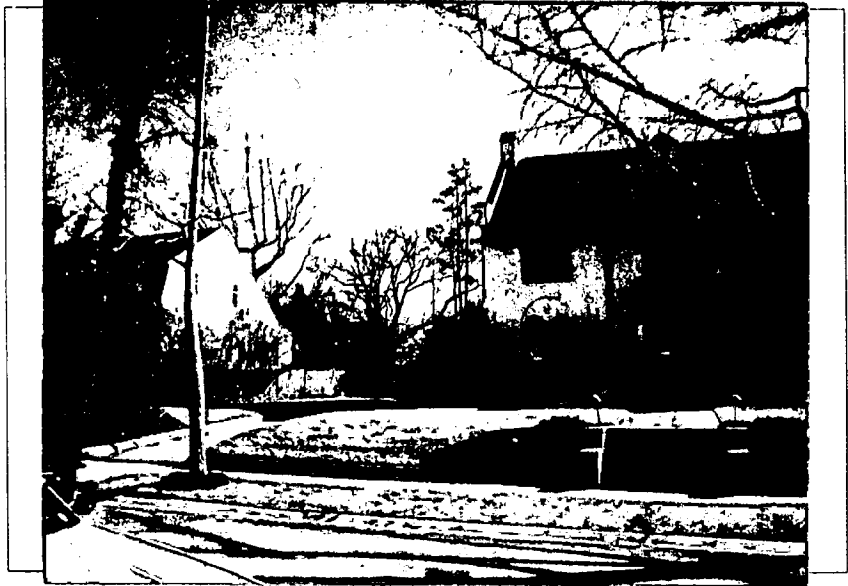
Detail: 20 end 16 Primrose Street from North West
