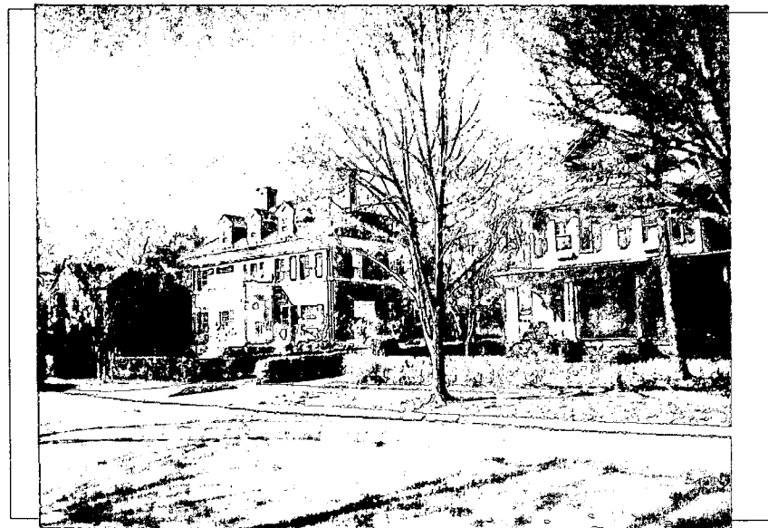
Detail: Primrose Street from #22 looking North West
