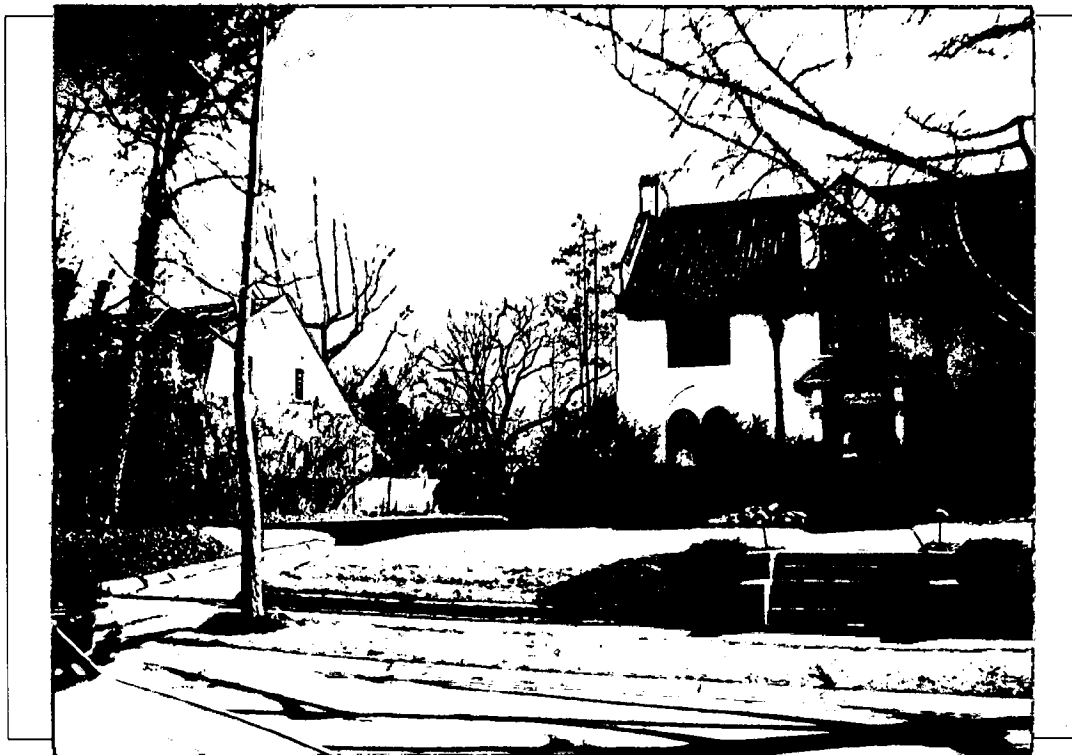
Detail: 22 end 16 Primrose Street from North West
