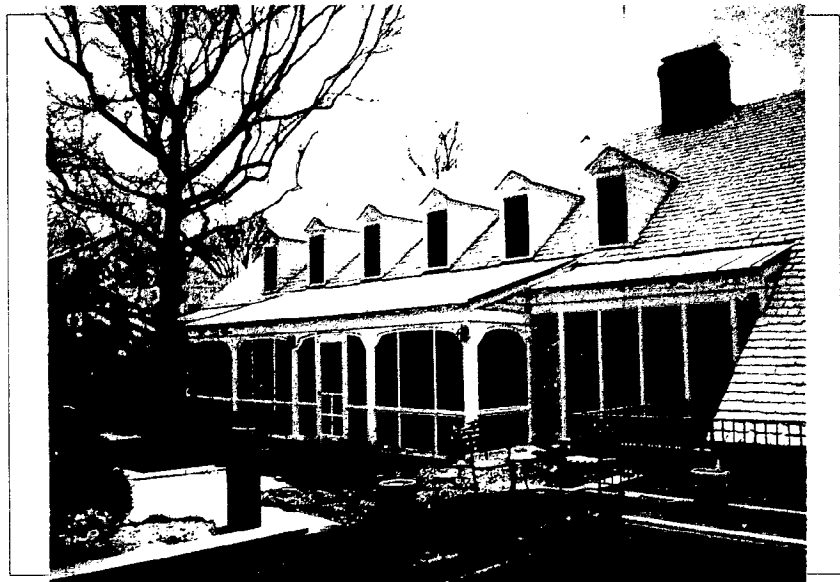
Detail: 22 Primrose St. (Rear) Close View From South East
