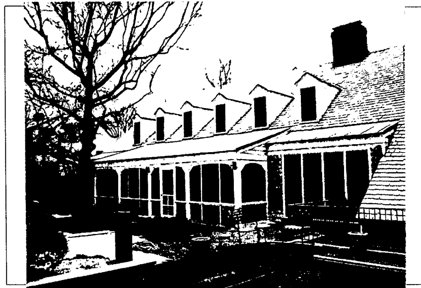
Detail: 22 Primrose St. (Rear) Close View from South East
