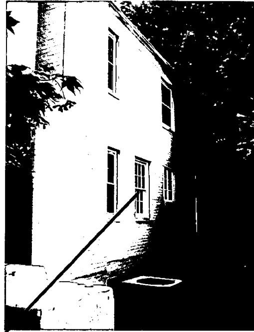
SIDE (EAST) ELEVATION NE
