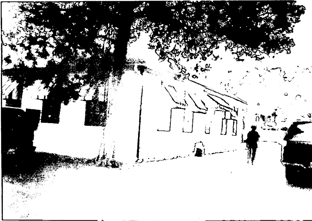
South facing 7201 Wisconsin Ave.
