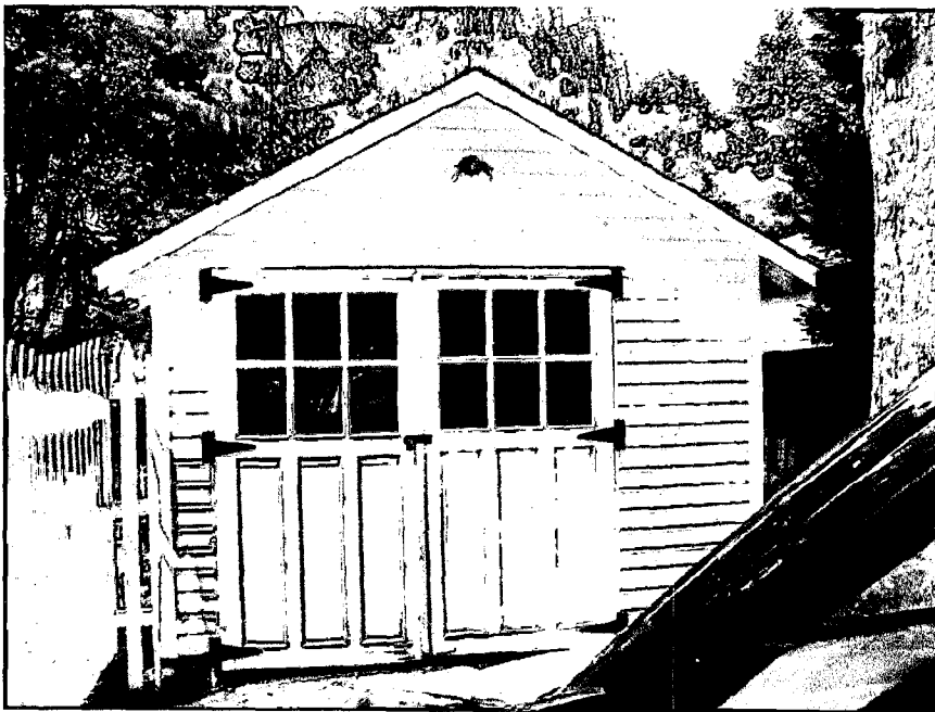
Garage with current rotting doors
