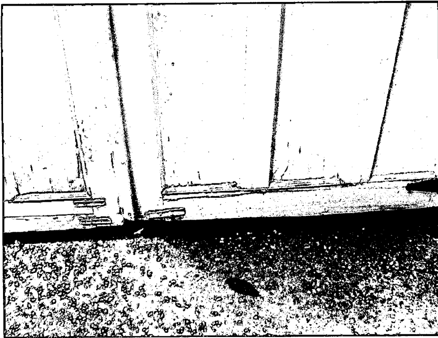
Close up of rotting wood. Note older repairs with metal brackets holding wood together.
