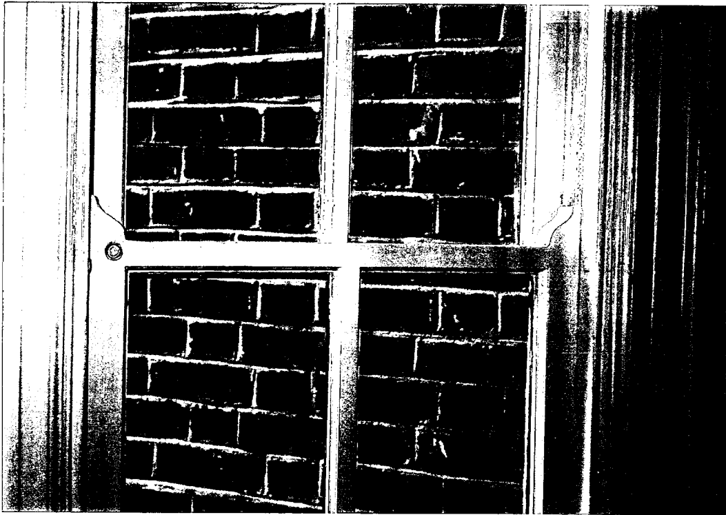
Photo #11: Interior detail view of meeting rail with tailpieces. Window No. 205.
