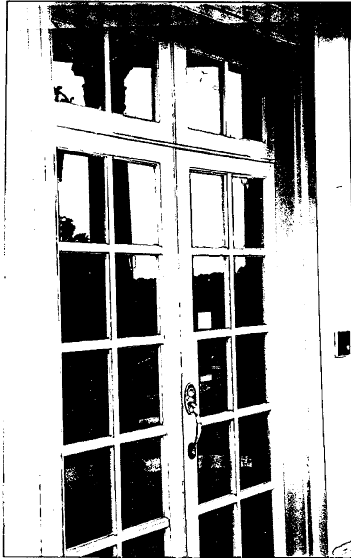
Photo #14: Exterior view of south entrance door No.s 109B. These doors will be replaced with new, double insulated French doors with egress hardware.
