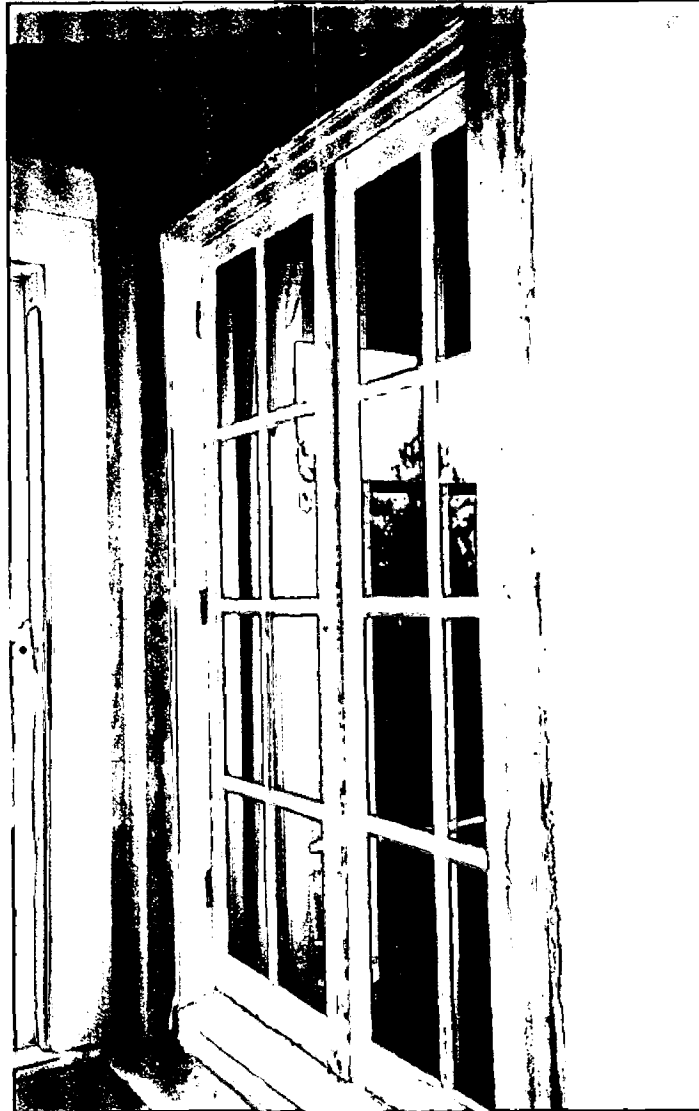
Photo #9: Detail view of exterior casement sash at Music Room. This sash opens onto the second floor hallway. This historic sash will be restored (archived) in place.
