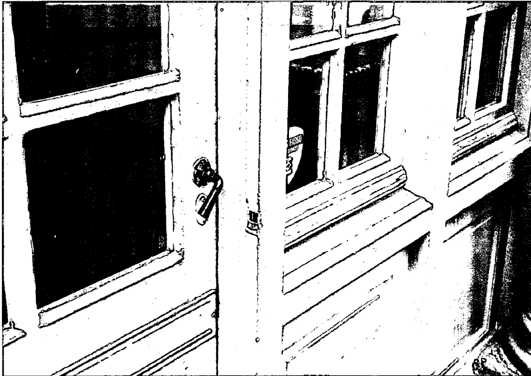
Photo #13: Detail view of window and door jambs at sun room. Exterior window mullions are already detailed (rabbeted) to receive exterior storm sash.
