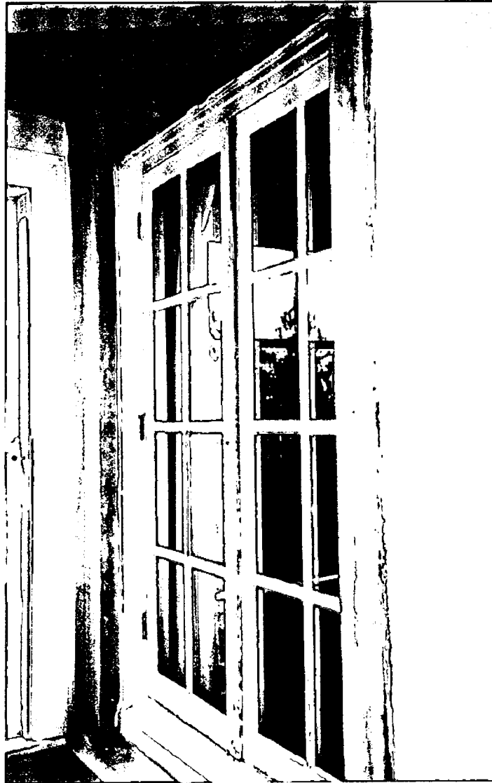
Photo #9: Detail view of exterior casement sash at Music Room. This sash opens onto the second floor hallway. This historic sash will be restored (archived) in place.
