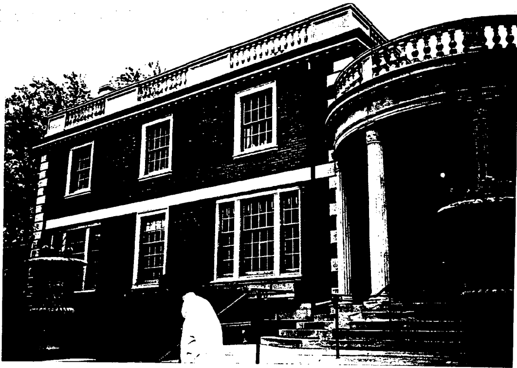
Photo #10: Exterior view of sash at first floor Gallery and kitchen, and second floor offices. The sash at the kitchen and offices must remain operable.
