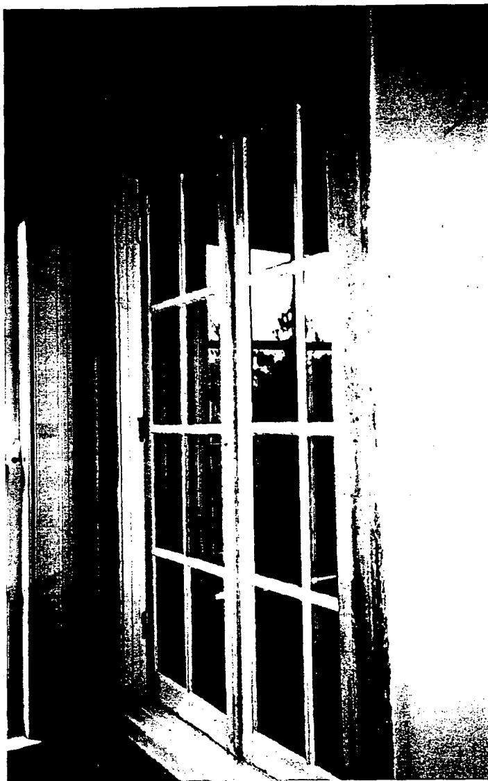
Photo #9: Detail view of exterior casement sash at Music Room. This sash opens onto the second floor hallway. This historic sash will be restored (archived) in place.
