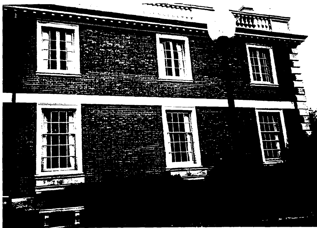
Photo #2: Exterior view of sash at Music Room.
