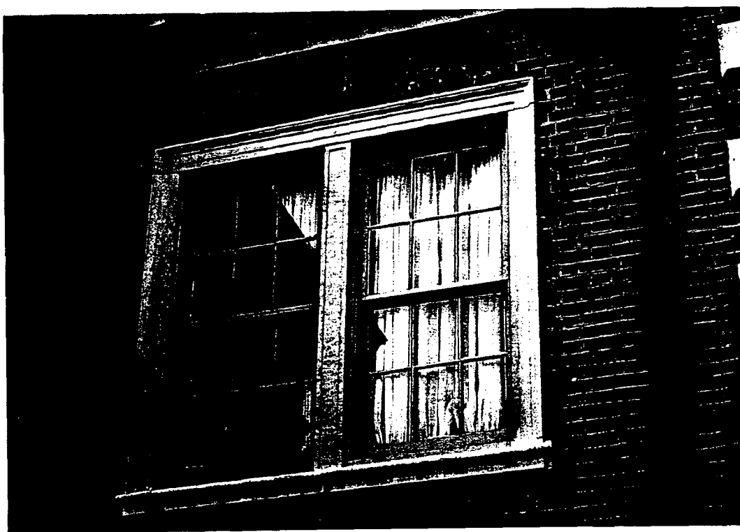
Photo #7: Exterior view of sash at second floor Gallery (Sash No.s 212, 213). Note narrow muntins (Type 3) at this sash.
