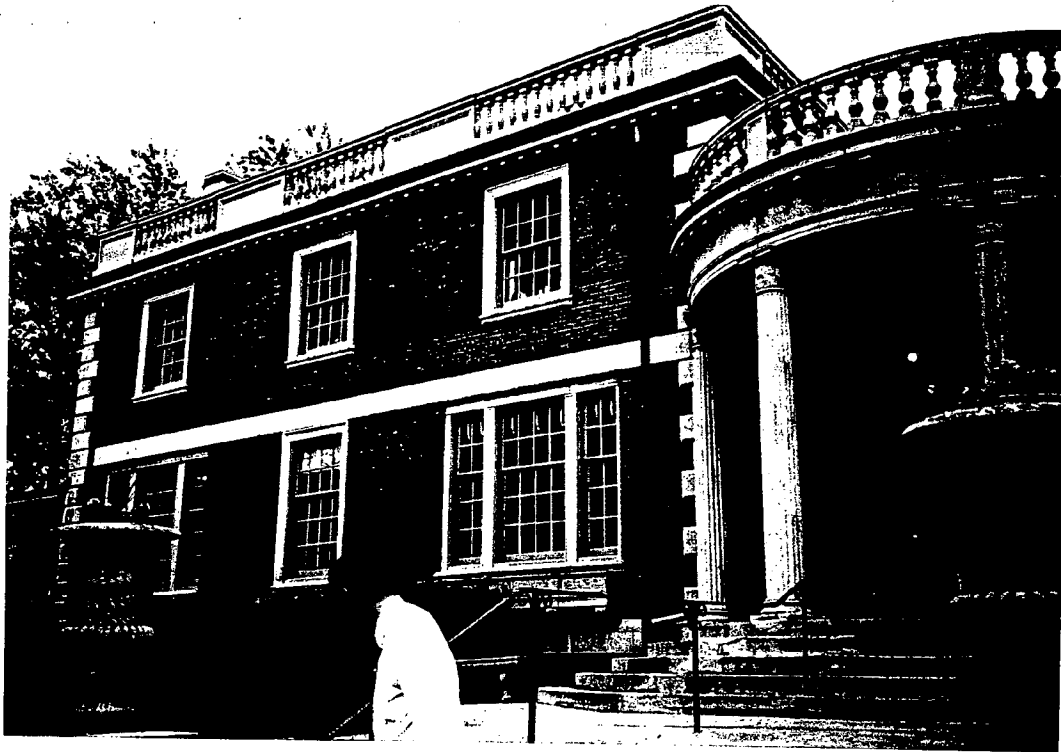
Photo #10: Exterior view of sash at first floor Gallery and kitchen, and second floor offices. The sash at the kitchen and offices must remain operable.
