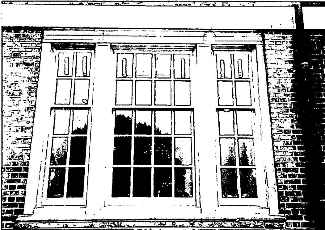
Photo #5: Exterior view of sash at Gallery (Rm. 110).
