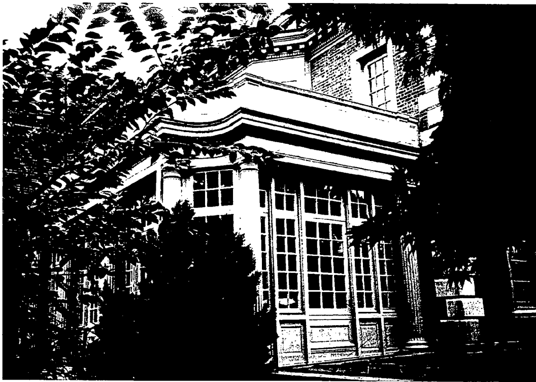
Photo #12: Exterior view of sun room window No.s 121 and 122. These sash will be restored and will receive exterior wood-framed storm glazing.
