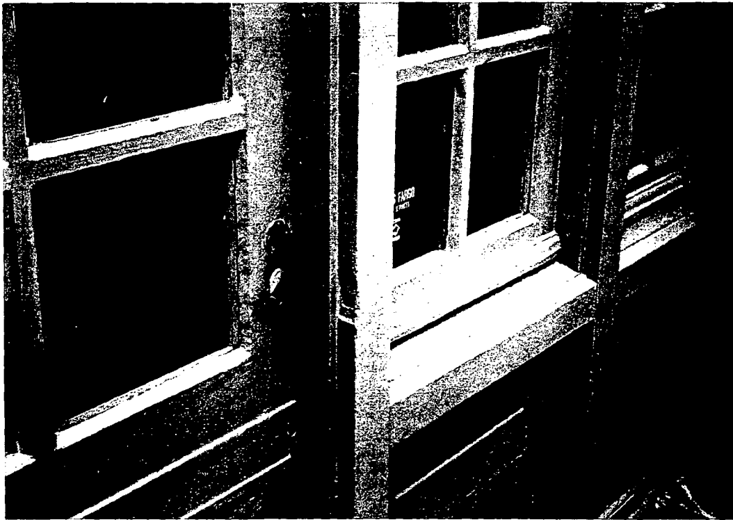
Photo #13: Detail view of window and door jambs at sun room. Exterior window mullions are already detailed (rabbeted) to receive exterior storm sash.
