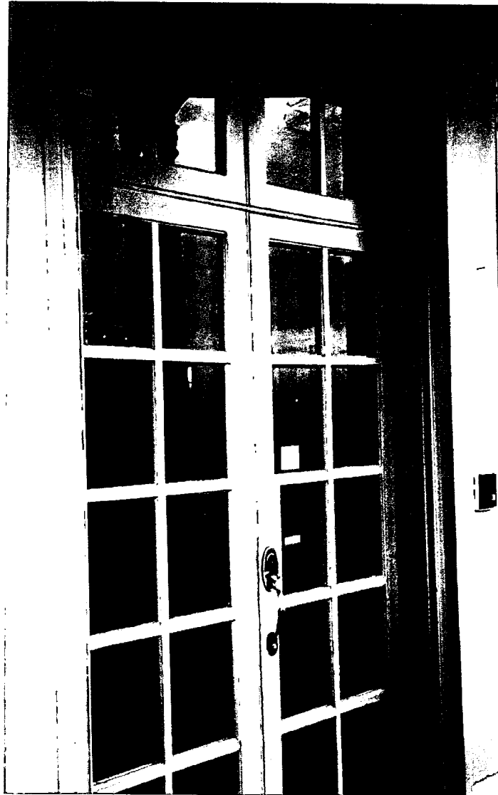
Photo #14: Exterior view of south entrance door No.s 109B. These doors will be replaced with new, double insulated French doors with egress hardware.
