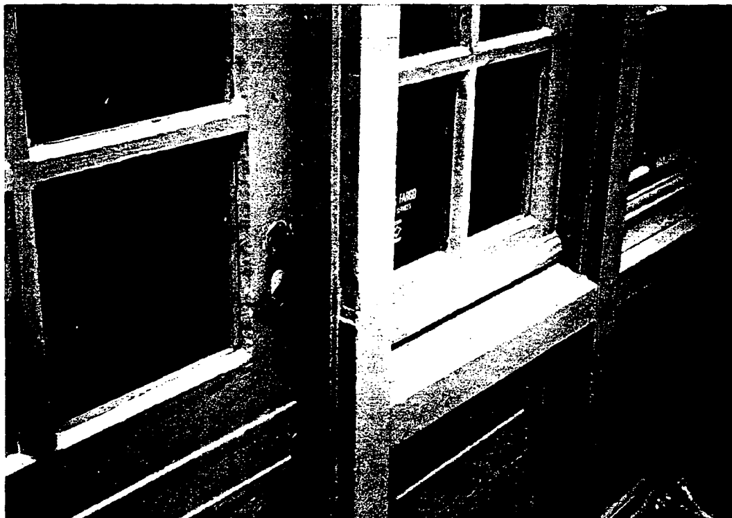
Photo #13: Detail view of window and door jambs at sun room. Exterior window mullions are already detailed (rabbeted) to receive exterior storm sash.
