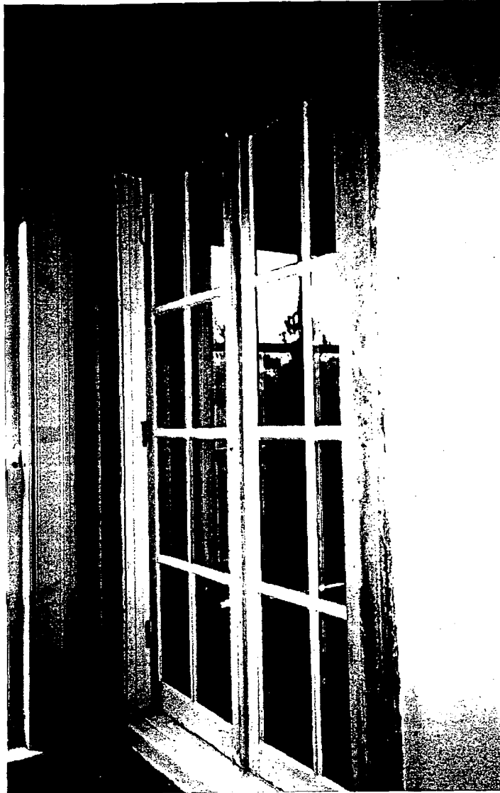
Photo #9: Detail view of exterior casement sash at Music Room. This sash opens onto the second floor hallway. This historic sash will be restored (archived) in place.
