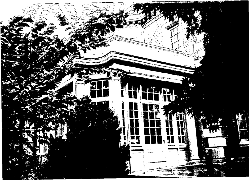
Photo #12: Exterior view of sun room window No.s 121 and 122. These sash will be restored and will receive exterior wood-framed storm glazing.
