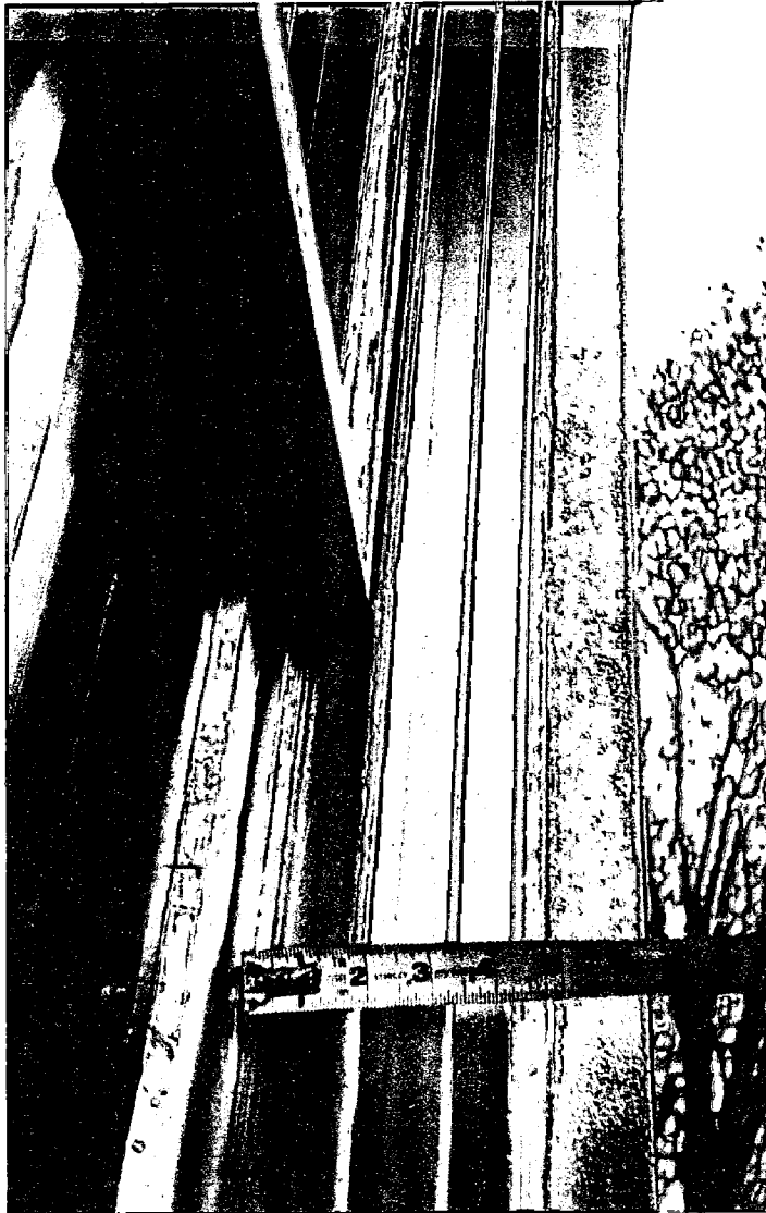
Photo #6: Detail view of jamb width for double-hung sash at first floor Gallery and Library. Window No.s 105 through 108.
