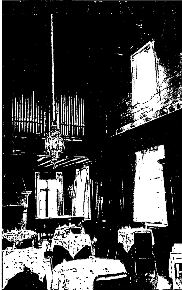
Photo #1: Interior view of music room. 8/12 Faux-finish double-hung sash are at lower level. 8x8 casement sash are at upper level.
