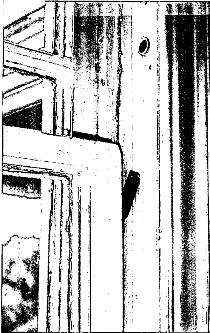
Photo #8: Detail view of loose sash at jamb (object easily fits in gap). This is a typical condition for all narrow-muntin sash at Strathmore Hall. See Photo #7 for exterior view of sash.
