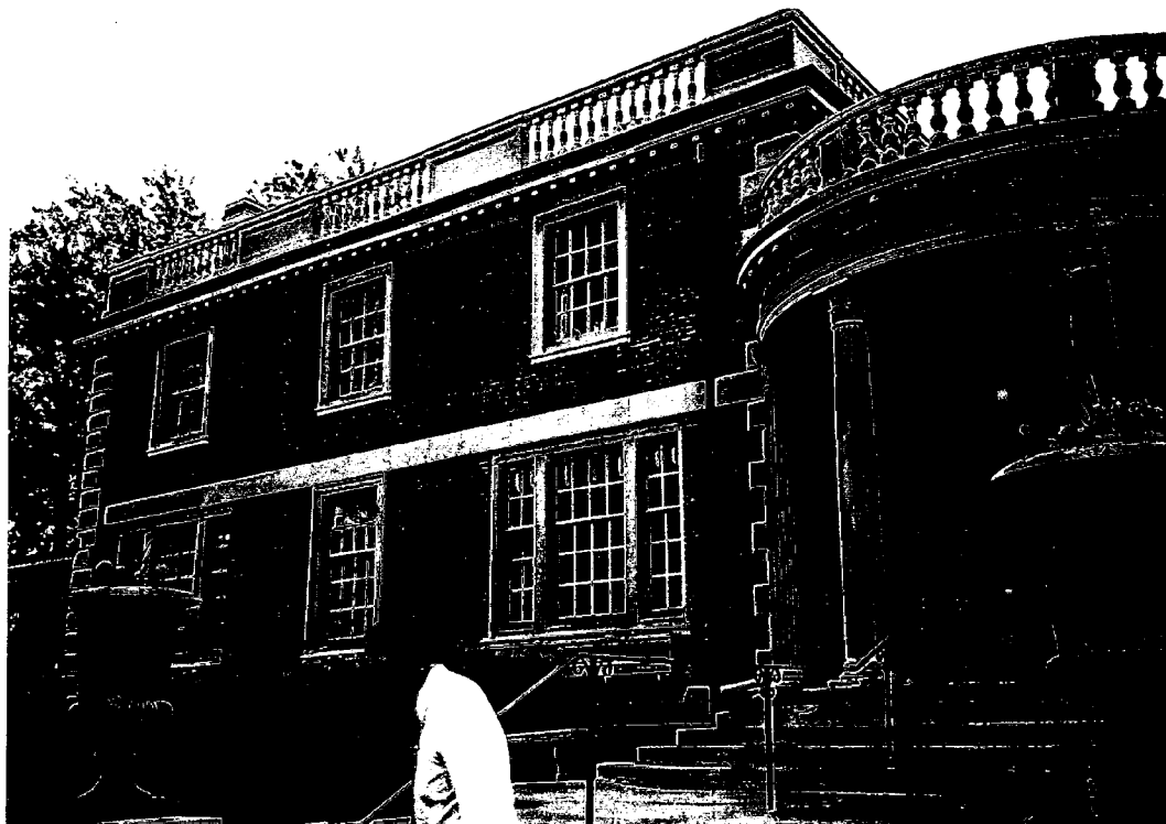
Photo #10: Exterior view of sash at first floor Gallery and kitchen, and second floor offices. The sash at the kitchen and offices must remain operable.
