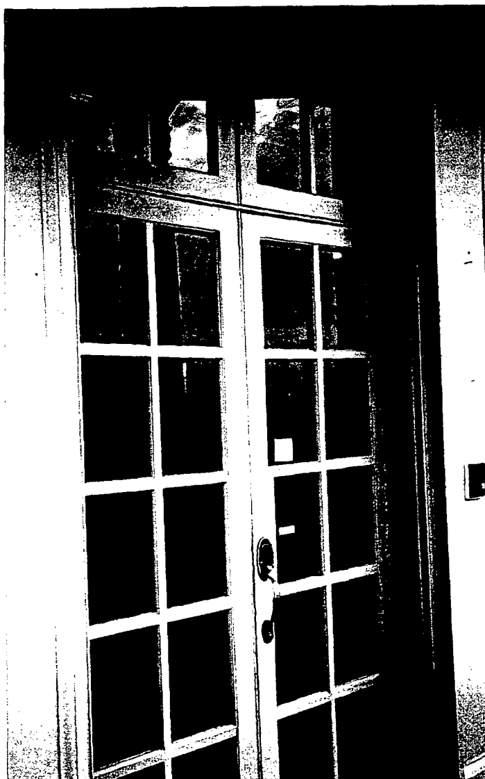
Photo #14: Exterior view of south entrance door No.s 109B. These doors will be replaced with new, double insulated French doors with egress hardware.
