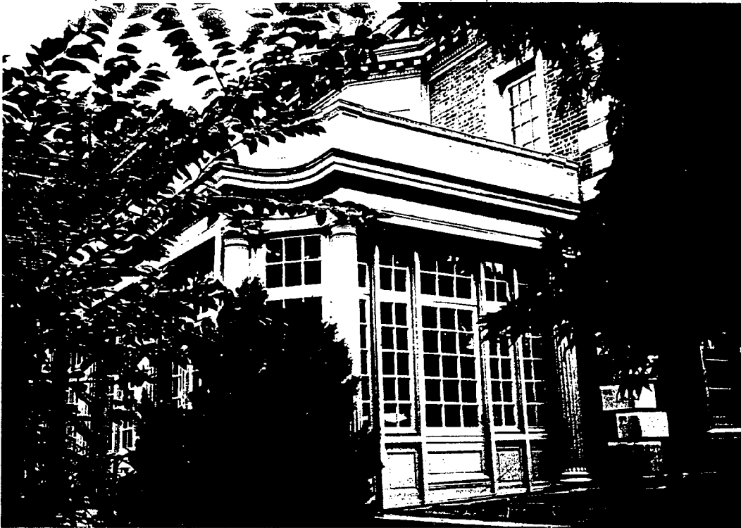
Photo #12: Exterior view of sun room window No.s 121 and 122. These sash will be restored and will receive exterior wood-framed storm glazing.
