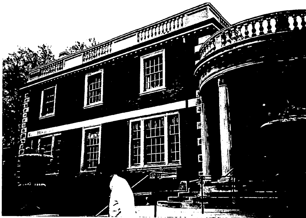
Photo #10: Exterior view of sash at first floor Gallery and kitchen, and second floor offices. The sash at the kitchen and offices must remain operable.
