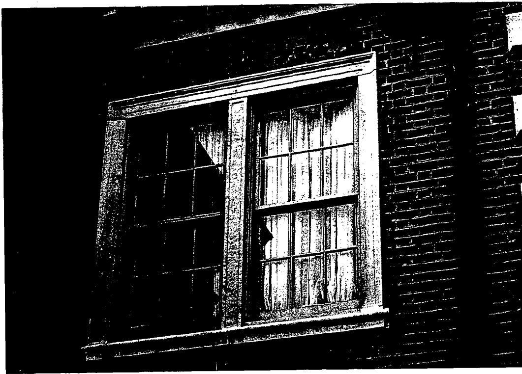
Photo #7: Exterior view of sash at second floor Gallery (Sash No.s 212, 213). Note narrow muntins (Type 3) at this sash.
