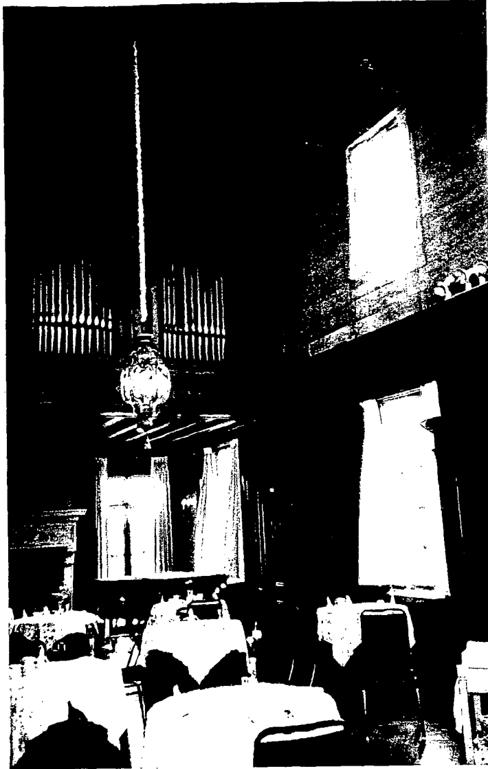
Photo #1: Interior view of music room. 8/12 Faux-finish double-hung sash are at lower level. 8x8 casement sash are at upper level.
