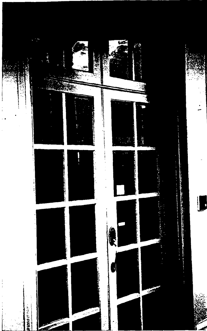
Photo #14: Exterior view of south entrance door No.s 109B. These doors will be replaced with new, double insulated French doors with egress hardware.
