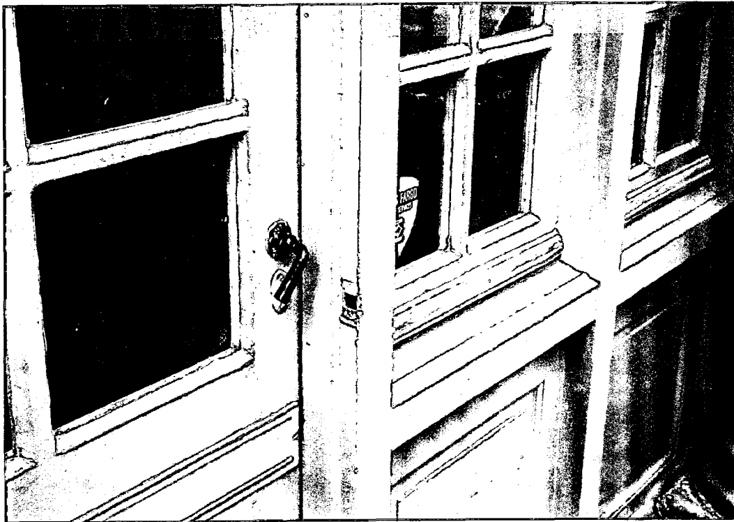
Photo #13: Detail view of window and door jambs at sun room. Exterior window mullions are already detailed (rabbeted) to receive exterior storm sash.
