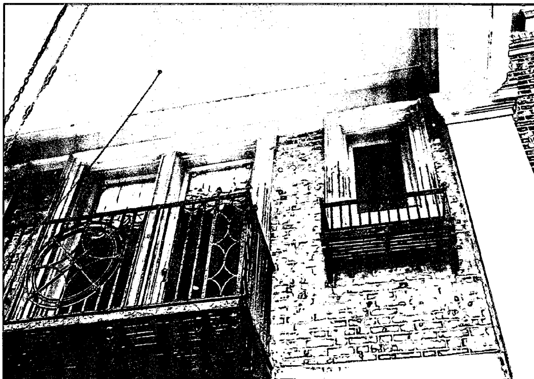
Photo #15: Exterior view of second floor French door No.s 259A. These doors will be replaced with true divided lite French doors.
