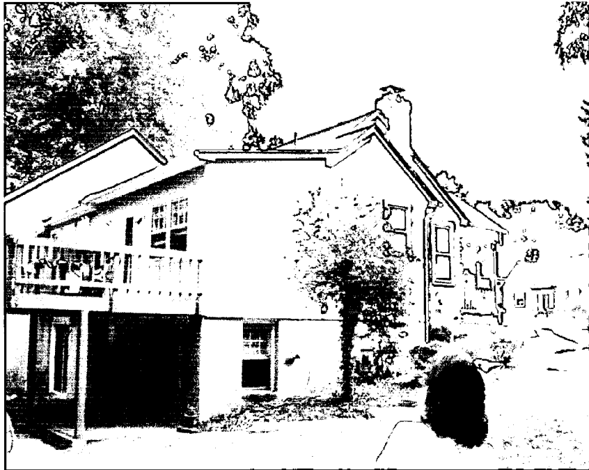
West Elevation - Rear Addition and Deck to be Removed; Original Gable to be Restored
