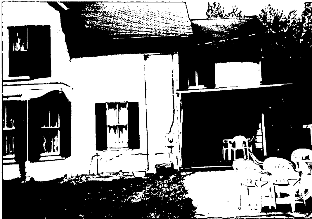
East Side of Structure - Open Porch - Proposed to be enclosed Windows same style + size as Existing Bay.
