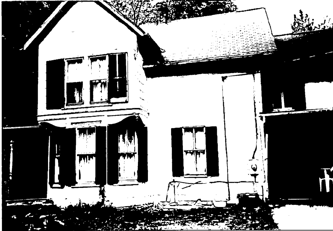
East Side of Structure
