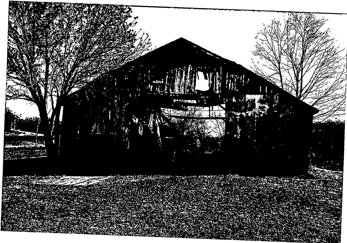
West elevation, looking east. Brewer Farm, Barn/Concrete Structure.
