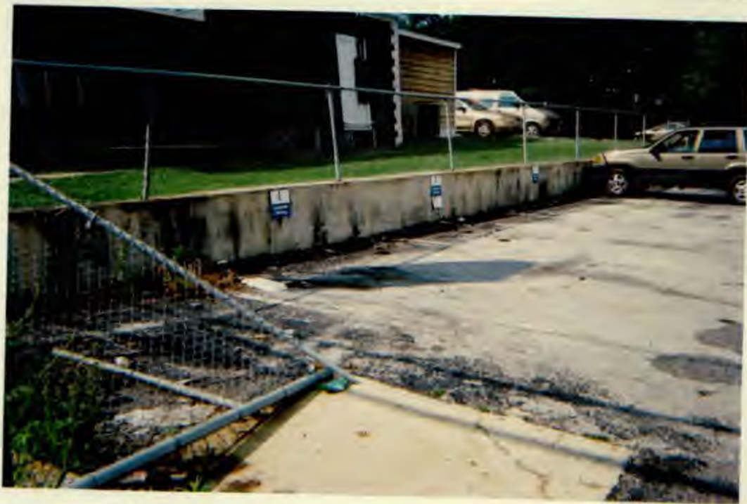
Front end of parking area and retaining wall.
