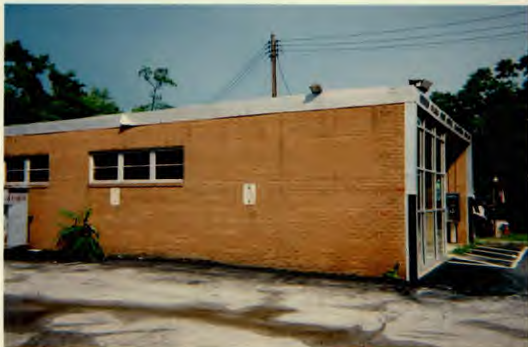
Front end of the North side of the building.
