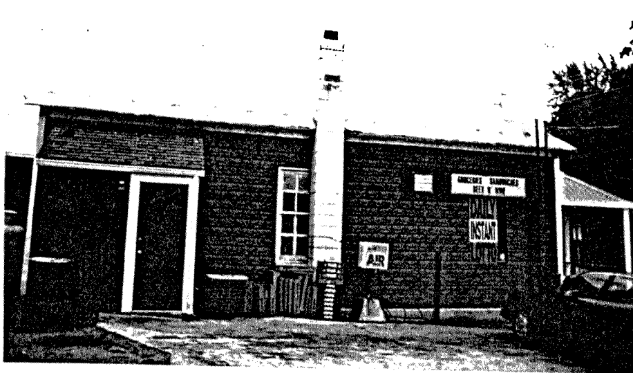
NORTH SIDE OF BLDG.
