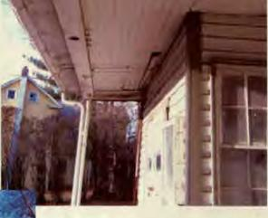
Front Porch, shows decay under gutter, steel posts.
