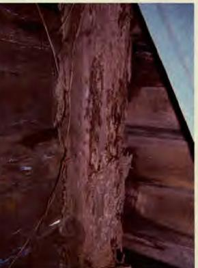
/North East corner, shows disconnected down spout and rotted gutter, facia, and siding.
