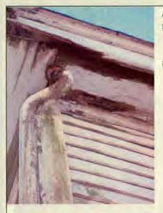
Exterior, shows extensive decay from disconnected down spout.
