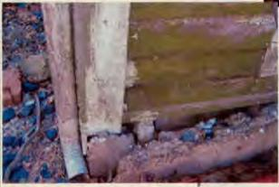
Foundation repair separating from foundation. Also shows moisture damage to siding.
